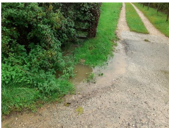
Blocked and hidden drains
