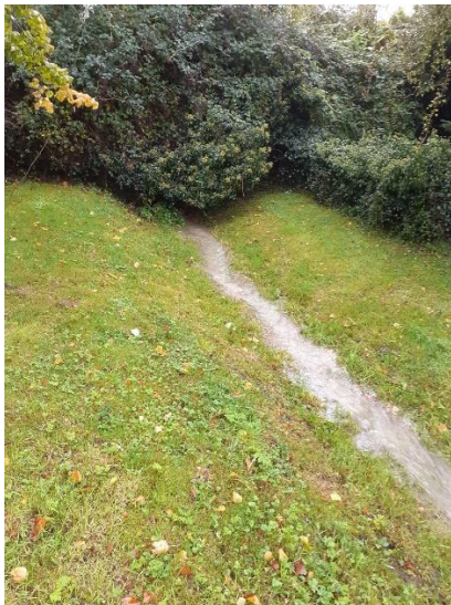
Blocked and hidden drains
