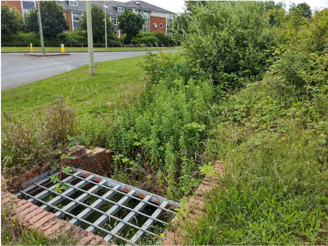
Plate 11 – Ditch, headwall and trash-screen adjacent to the gate in the south-east
