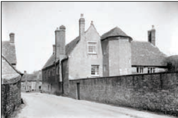
View along Church Lane with Manor House to the right, with its hexagon stair tower (Packer Collection - Simms 191 - 40). The rear of the Manor house remains although
