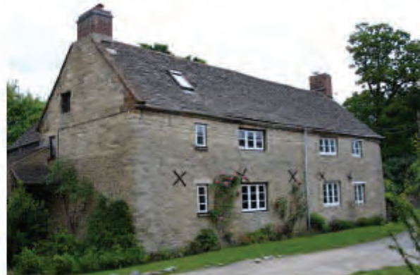
4 and 5 Southend Cottages
