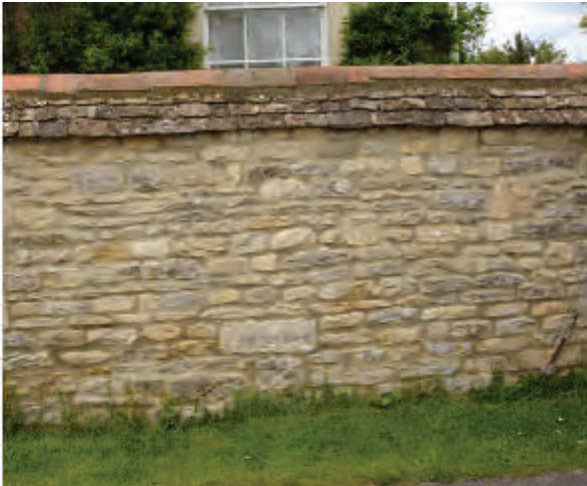
Tiles and stone slates form coping
