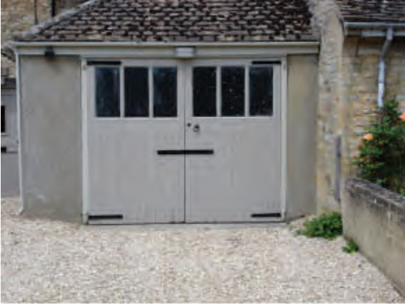
Vertically hung timber garage doors.
