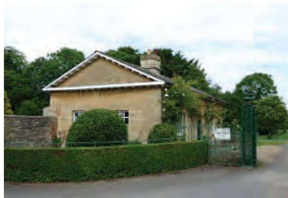
North entrance lodge to Kirtlington Park.
