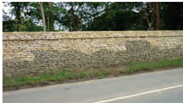
Kirtlington Park boundary wall on Heyford Road
