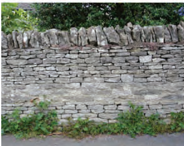
Stone laid on edge forms coping
