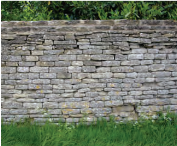
Mortared stone course forms coping
