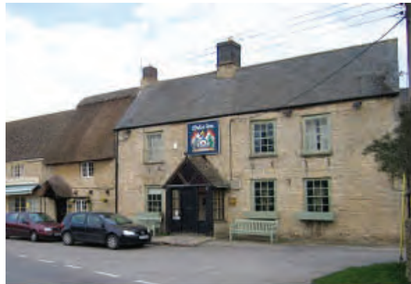
The Oxford Arms Public House and Cottage.
