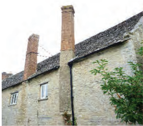
External chimney at the Manor House
