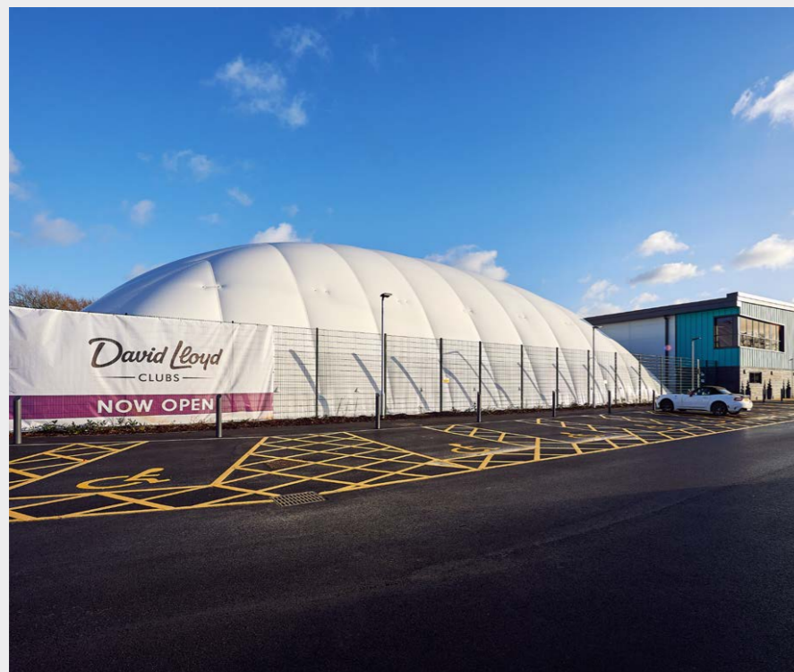
Fig.16 External of typical airdome
