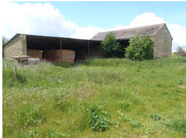
Barns in western part of site
