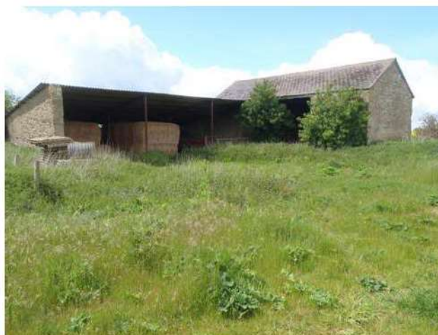
Barns in western part of site
