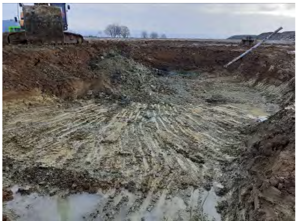
09.02.21 – Removal of impacted soils until visual, olfactory indicators absent and low (<10ppm) readings recorded on PID. Base of excavation in northeast onto clay.
