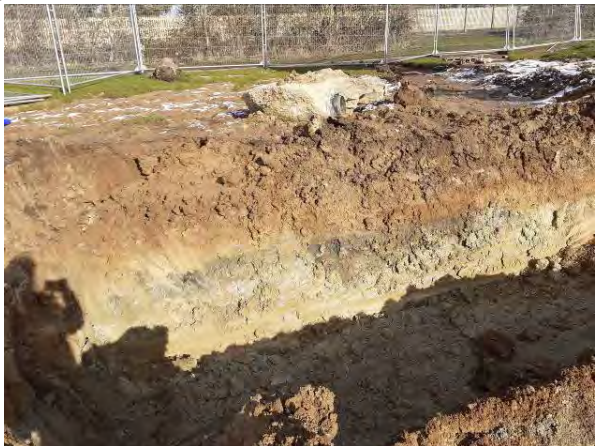
09.02.21 – Northern sidewall of remediation excavation absent of any significant contamination indicators suggesting sufficient removal of impacted soils
