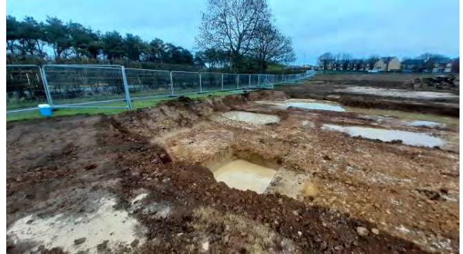
14.01.21 – Eastern view across the hotspot area with partial recovery of clean surface soils and a series of trial-pits / trenches to delineate extent
