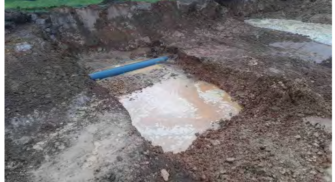
14.01.21 – Exposure of POL pipeline in the north. Shallow ingress of groundwater, no sheen, floating product or globules observed.
