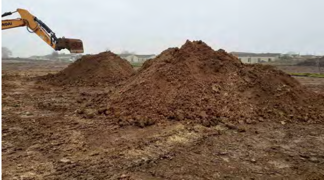
14.01.21 – Clean soils temporary stockpiled on surface to allow inspection prior to relocation to temporary holding area
