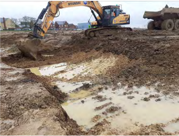
02.02.21 – Excavation of clean overlying soils and removal from remediation area to allow extension down to impacted soils
