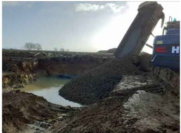
03.02.21 – Backfill of remediation excavation with aggregates
