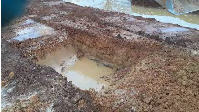
14.01.21 – Excavation of a series of shallow trial-pits to delineate extent of impacted soils
