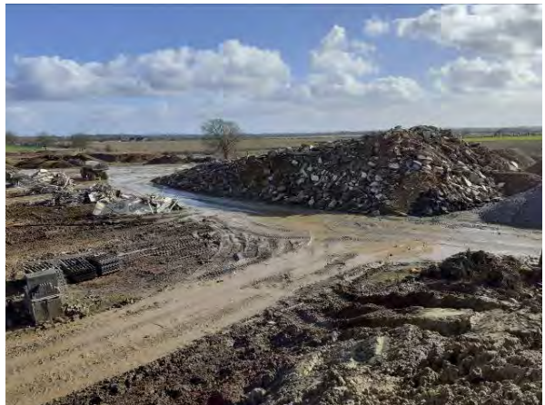
16.02.21 – Stockpile of recovered hardstanding prior to processing
