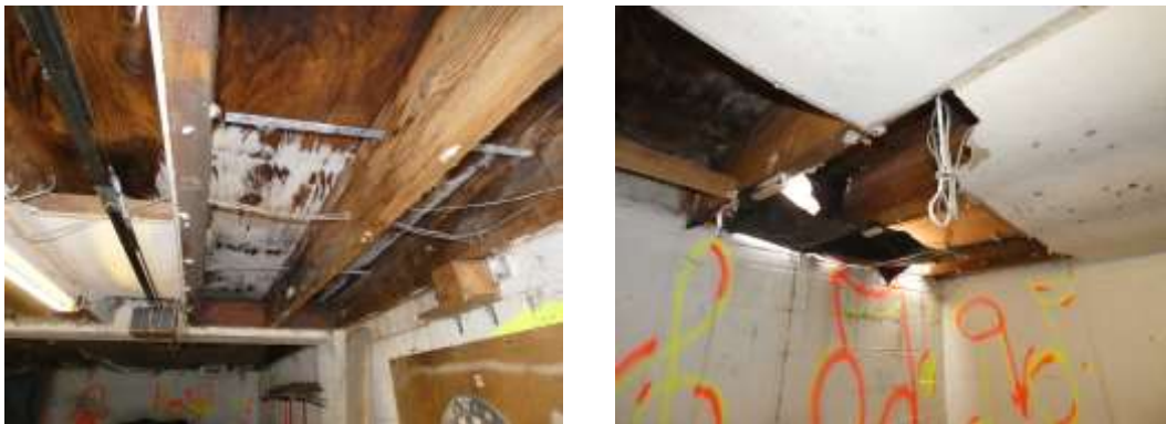
Figs. 13 & 14 Interior of garage
