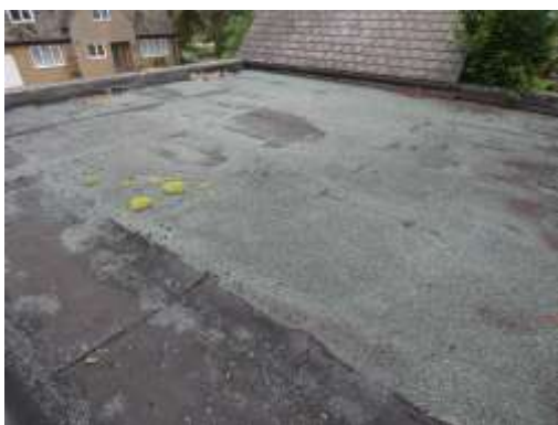
Figs. 5 & 6 Felt covered roof of garage
