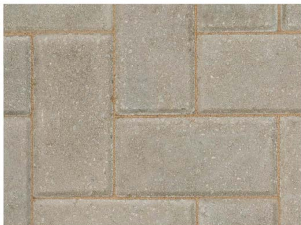
03 027 BLOCK PAVING TO CAR PARK CIRCULATION natural
