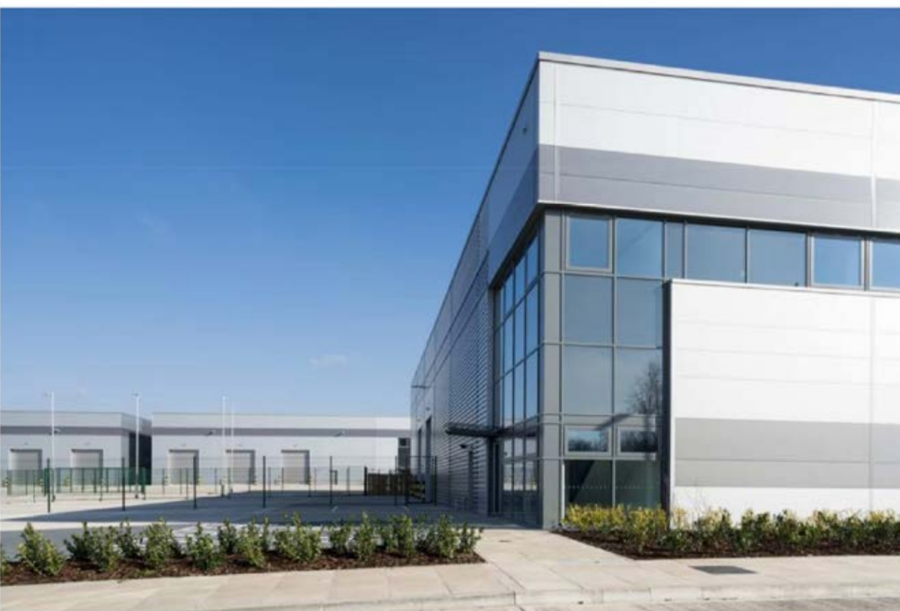
11 027 COMPOSITE PANEL FACADE AND CURTIAN WALLING (top down) Micro lined composite panel facade example
