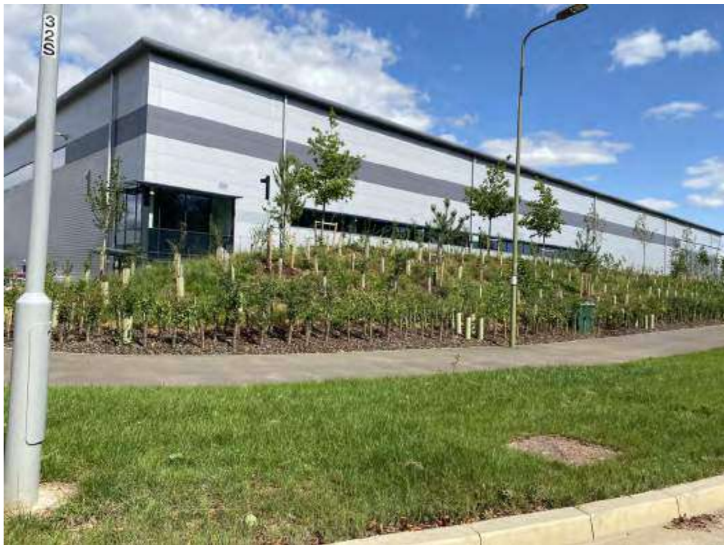
Fig. 07 Unit 1 Phase 1 viewed from Middleton Stoney Road
