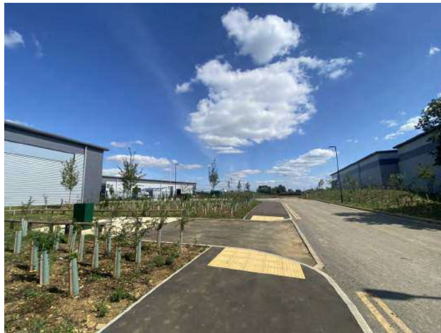
Fig. 06 Looking South East on temporary initial road
