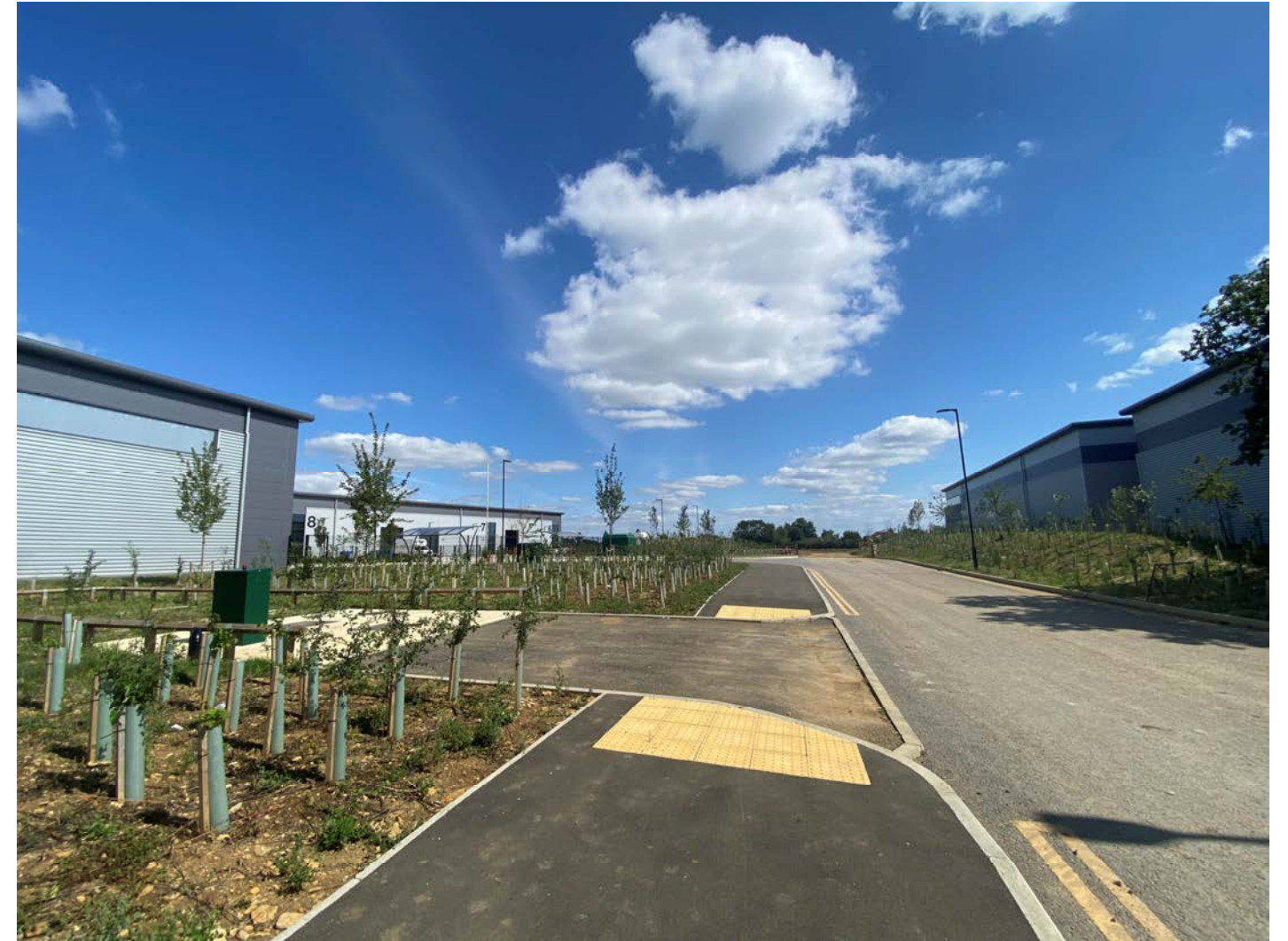
Fig. 06 Looking South East on temporary initial road
