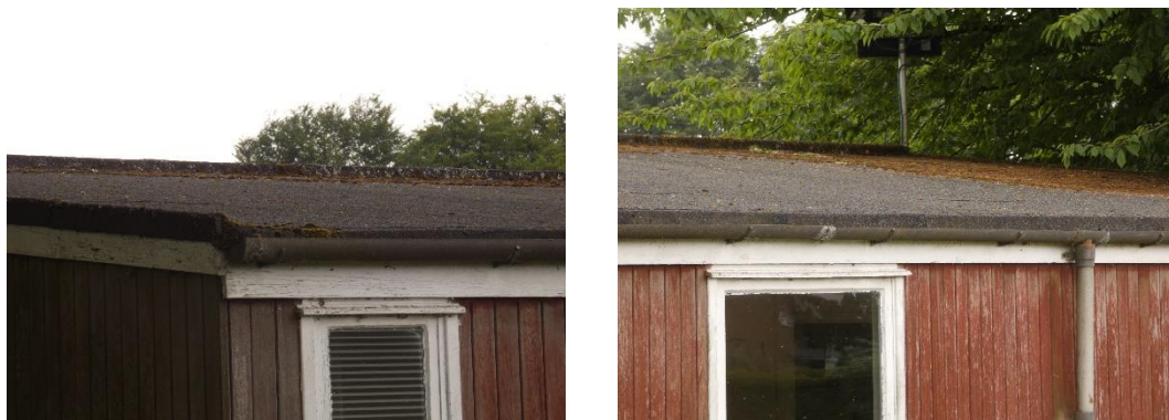
Figs. 3 & 4 Roof felt un-torn
