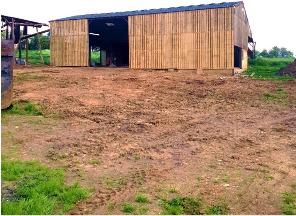
Figure 1 – Existing Southern Elevation of Application Building
