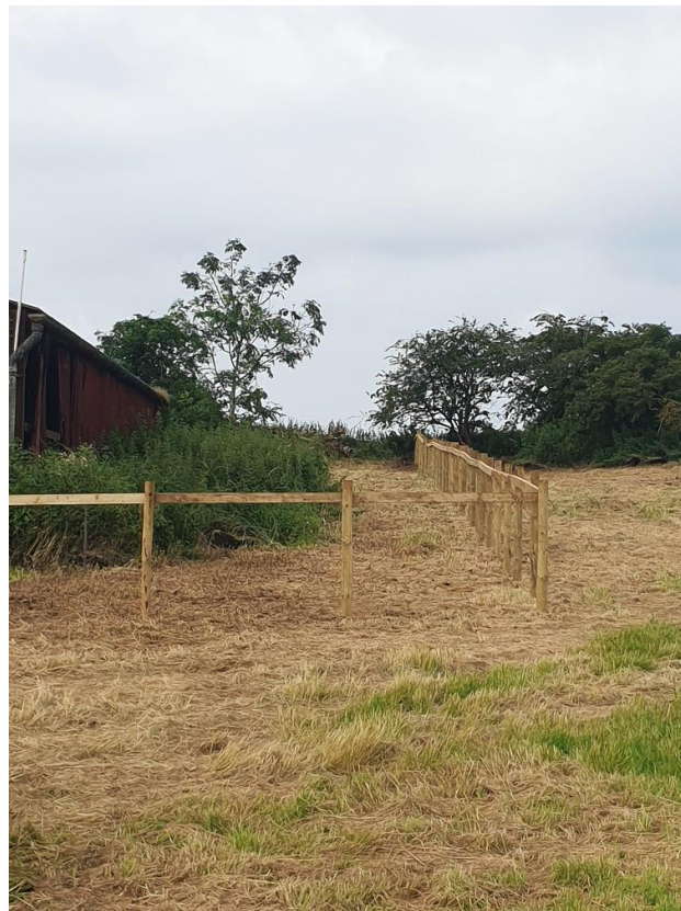
Figure 3 – Fencing on site (north)
