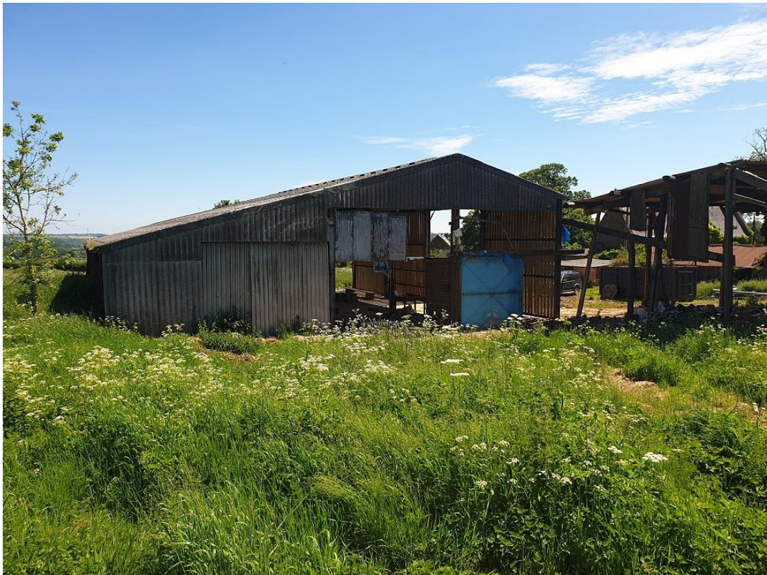
Pole barn part demolished
