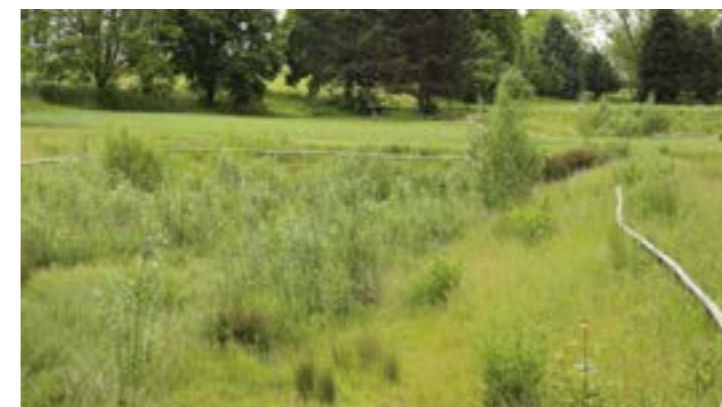
PLANTED ATTENUATION BASIN
