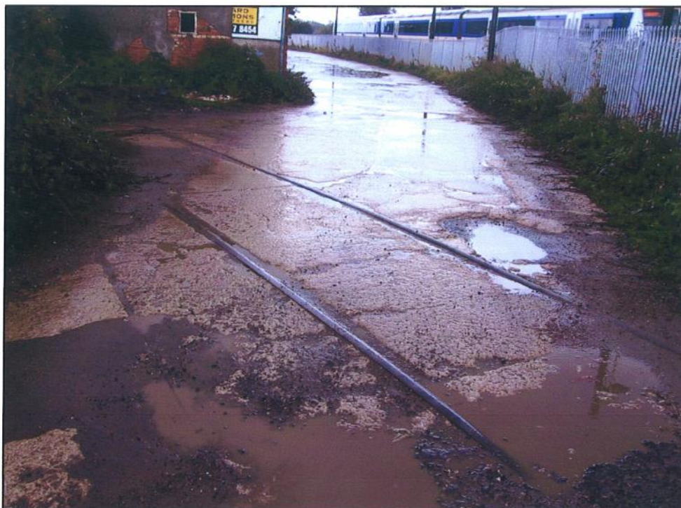
Plate 8: Redundant railway lines entering site.
