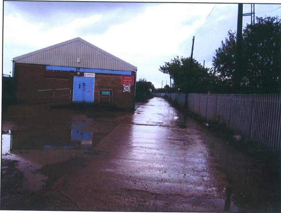
Plate 9: Access road along site boundary.
