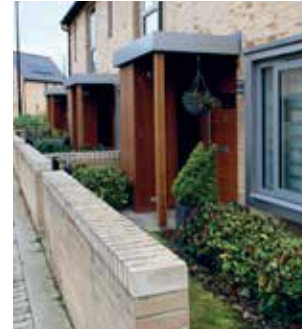
Front boundary wall with planting behind
