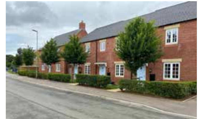
Victoria Park: Consistent building line and low hedgerow to front boundary treatment
