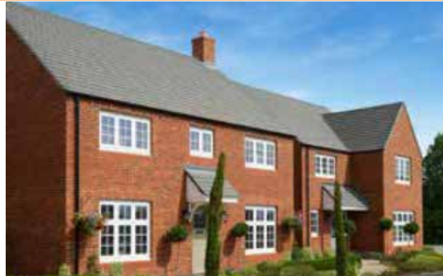
Bloxham Vale: Predominance of red brick and grey tiles. detailing including porches and chimneys
