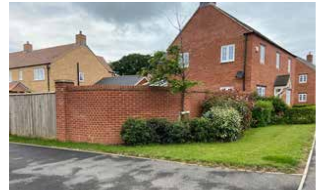
Bloxham Vale: 1.8 m brick wall to match house materials
