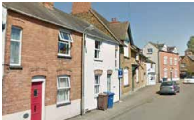
Banbury: Variation in roof profiles. Use of brick detailing to windows. Mix of textured red brick, stone and render. Predominantly grey tiles.
