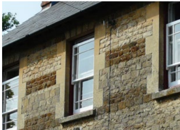
Timber frame sash glazing with limestone ashlar jambs
