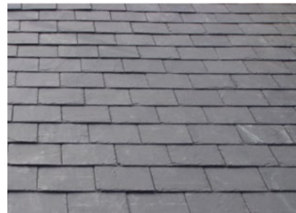
Welsh slate roof
