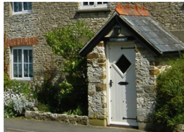
Timber panel door
