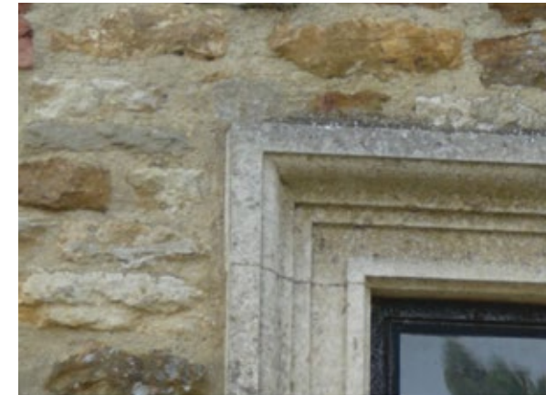
Coarse Limestone stone with Limestone Ashlar Window Reveal
