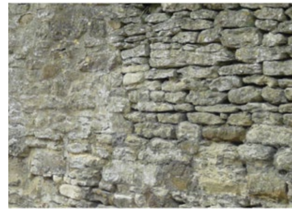
Rubble Limestone of a boundary wall
