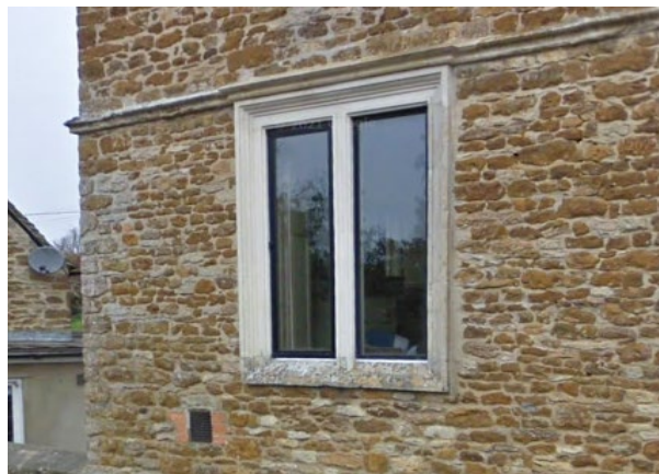
Metal window with carved limestone reveal
