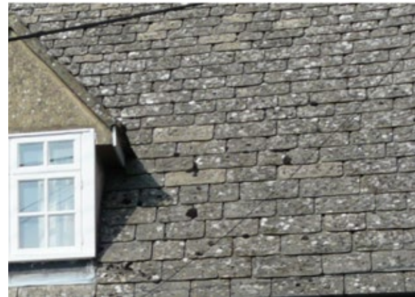
Stonefield slate roof
