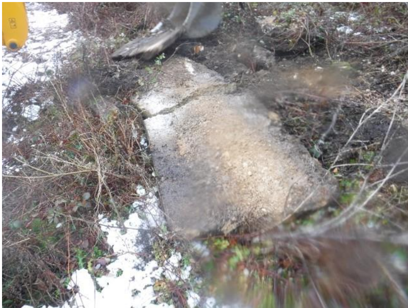
Limited concrete slab near to caravan base
