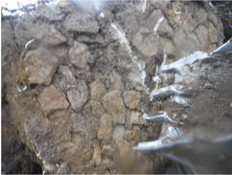
Underside of Concrete Slab
