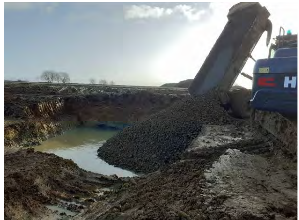
03.02.21 – Backfill of remediation excavation with aggregates
