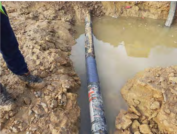
03.02.21 – POL pipeline exposed in the northwest. Wrapping around pipework suggests possible historical repair work
