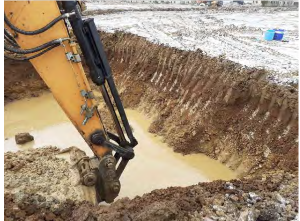
08.02.21 – Recovery of clean overlying soils from hotspot area. Ingress of shallow groundwater, no sheen, globules or floating product observed.
