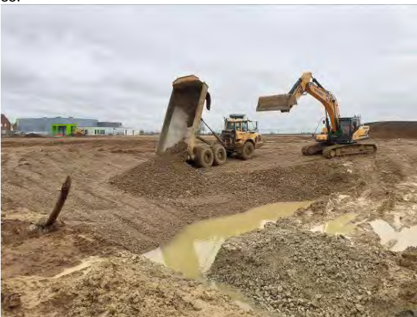
16.02.21 – Backfilling of remediation excavation with aggregate concurrently with removal of impacted soils
