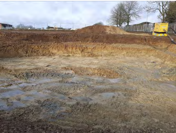
17.02.21 -. Completed extent of remediation excavation in the north / northwest. Base and sidewalls ready for validation samples to be collected
