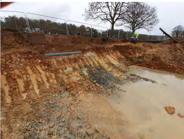
17.02.21 - Residual pocket of impacted soil awaiting removal
