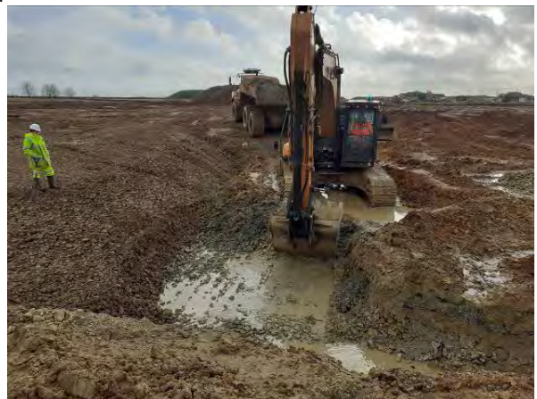
16.02.21 – Removal of impacted soils down to bedrock. Ingress of groundwater at surface of bedrock, no sheens observed.
