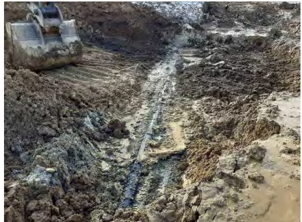
09.02.21 – Exposure of POL pipeline which ran north to south through the centre of the baseball pitch
