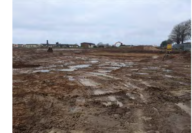
02.02.21 – View across baseball pitch following stripping and recovery of topsoil
