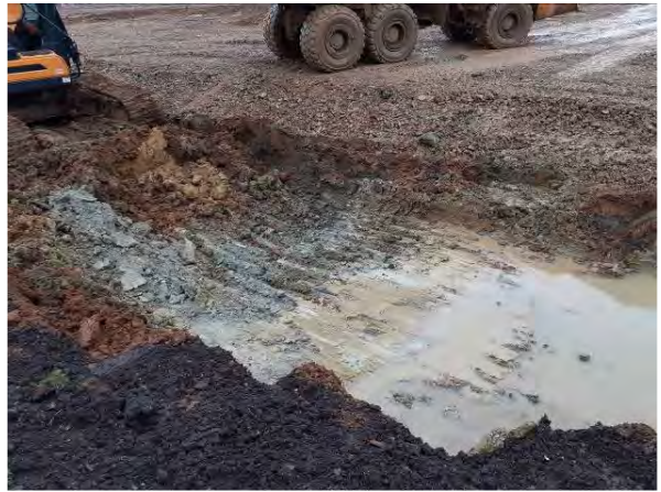
18.02.21 – Removal of impacted soils down to layer of clean clay above shallow bedrock
