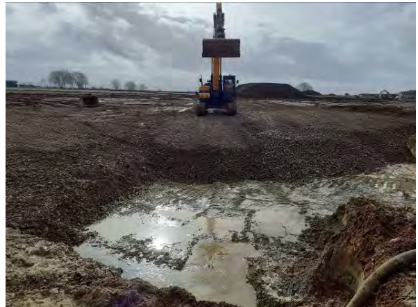
17.02.21 - Backfill of remediation excavation immediately following the collection of samples due to the ingress of groundwater
