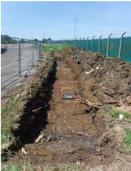
Trench 1. NW View
