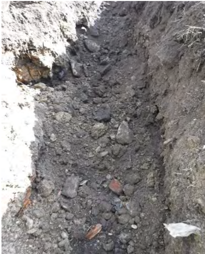
Trial Trench TP16
