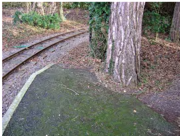
Photograph 11 – The base of Pine tree T69 against the back of the raised platform.
