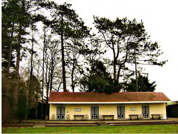
Photograph 10 – Pine tree T69 to the left of picture and Yew tree T79 to the far right behind the station pavilion building.
