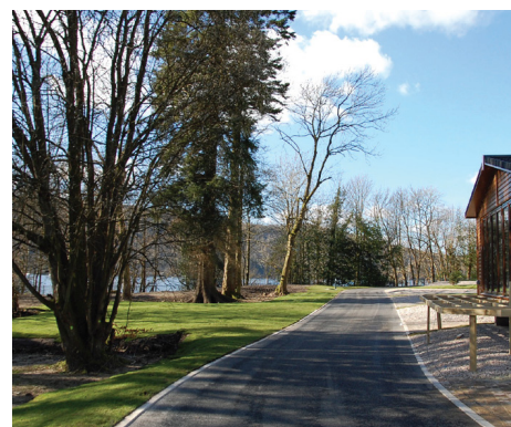
Fallbarrow Park, Windermere: Completed CellWeb TRP® Installation
