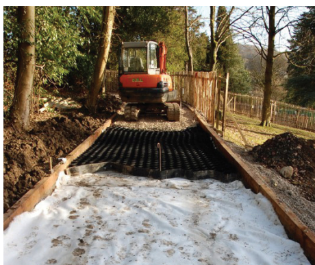
Fallbarrow Park, Windermere: CellWeb TRP® Installation
