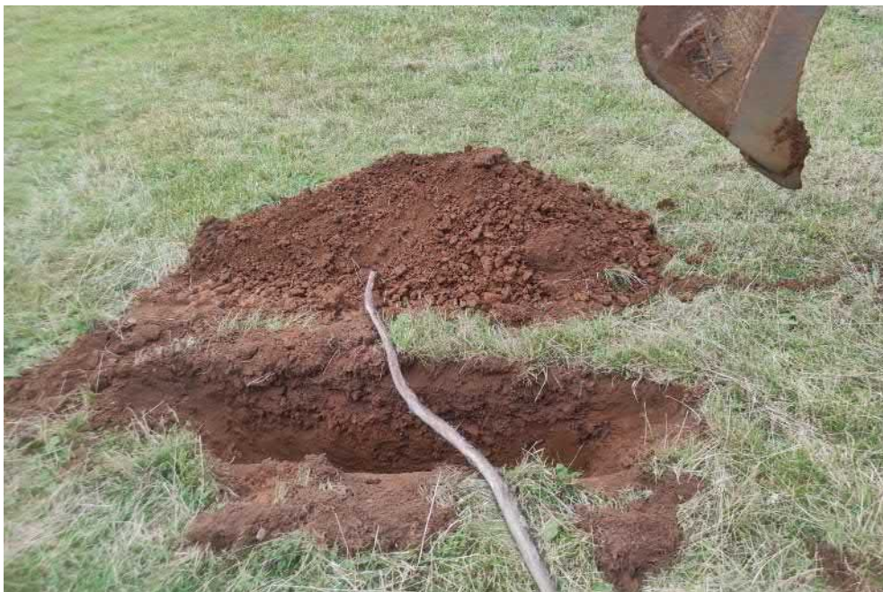
Photograph of arisings from trial pit SA8.
