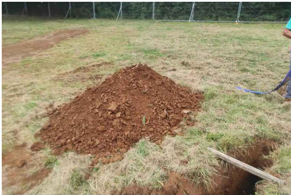
Photograph of arisings from trial pit SA5.
