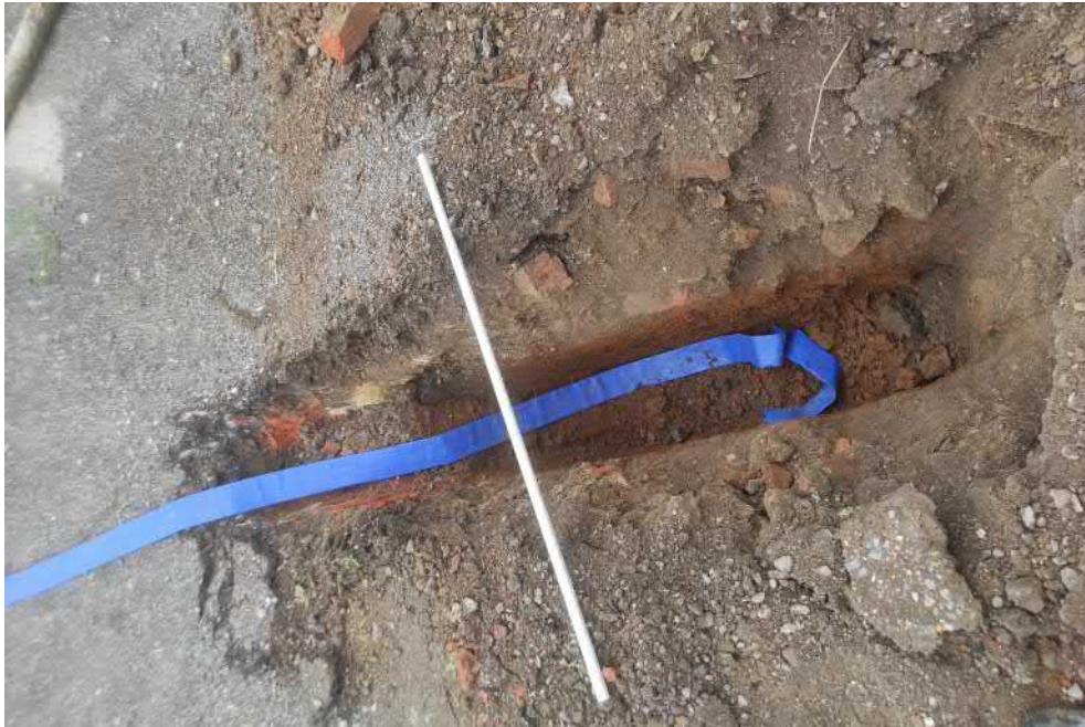
Photograph of trial pit SA1.
