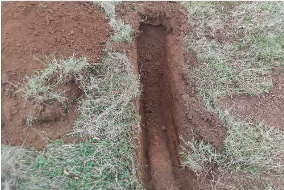
Photograph of trial pit SA7.
