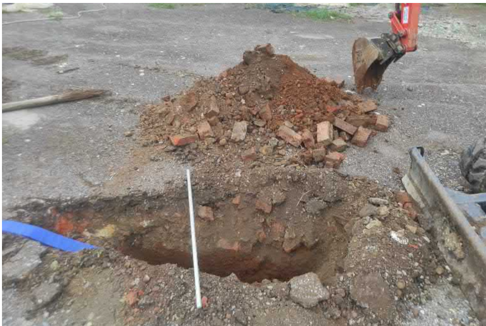
Photograph of arisings from trial pit SA1.
