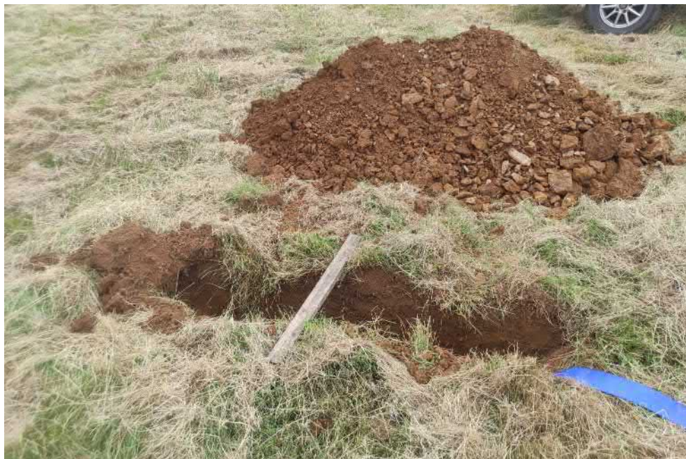
Photograph of arisings from trial pit SA4.
