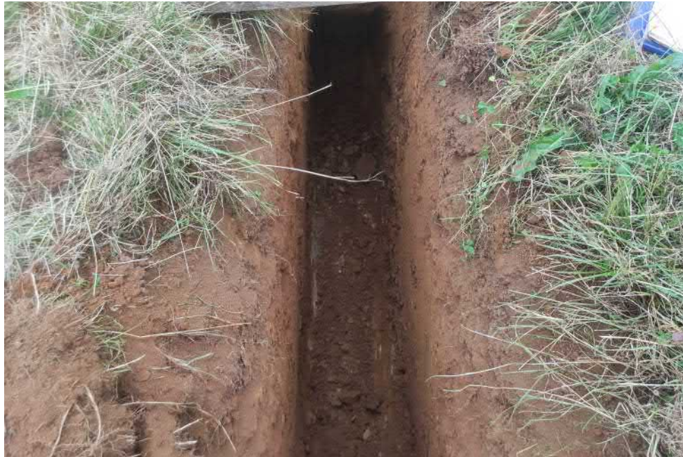
Photograph of trial pit SA5.
