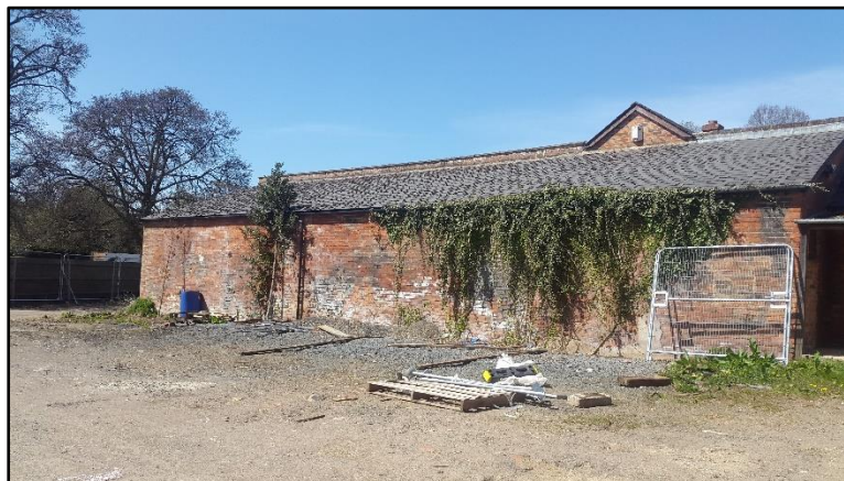
Plate 3: Showing B1. Photograph looking west.
