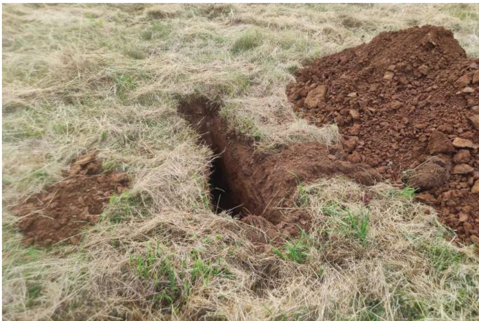
Photograph of arisings from trial pit SA3.
