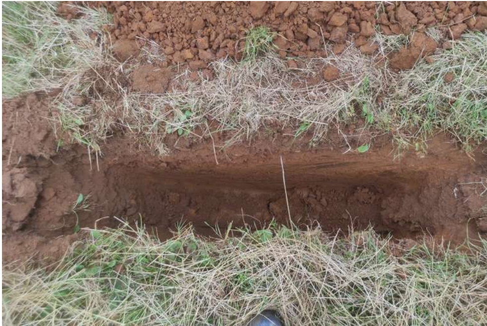
Photograph of trial pit SA2.
