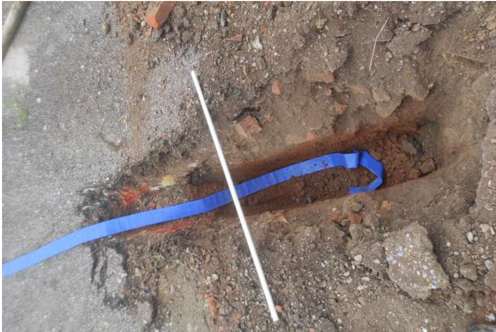
Photograph of trial pit SA1.
