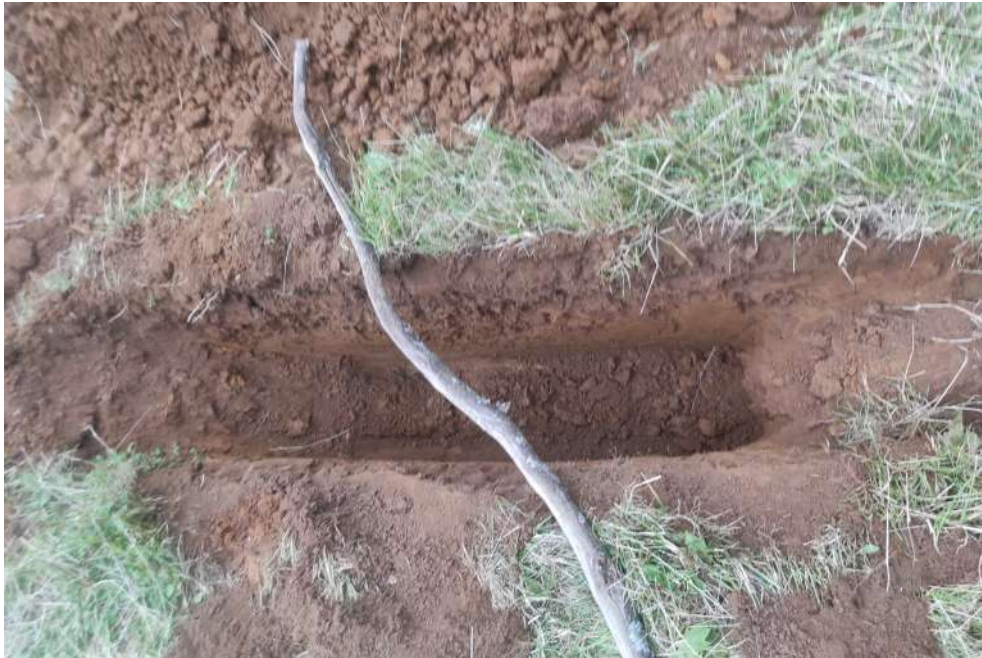
Photograph of trial pit SA8.
