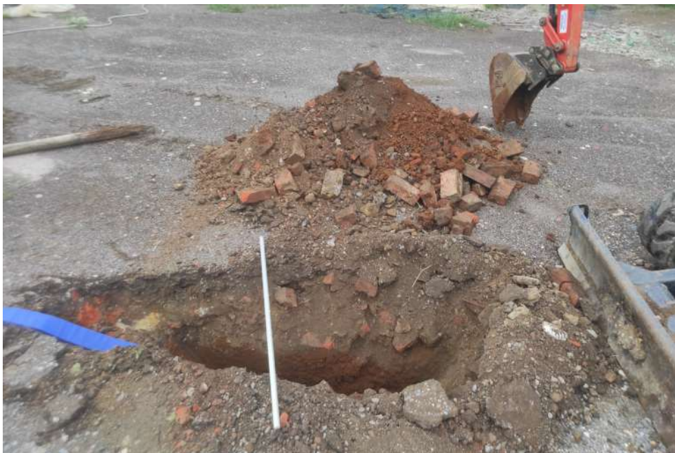
Photograph of arisings from trial pit SA1.
