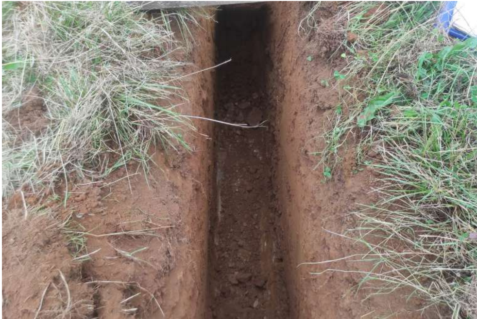
Photograph of trial pit SA5.
