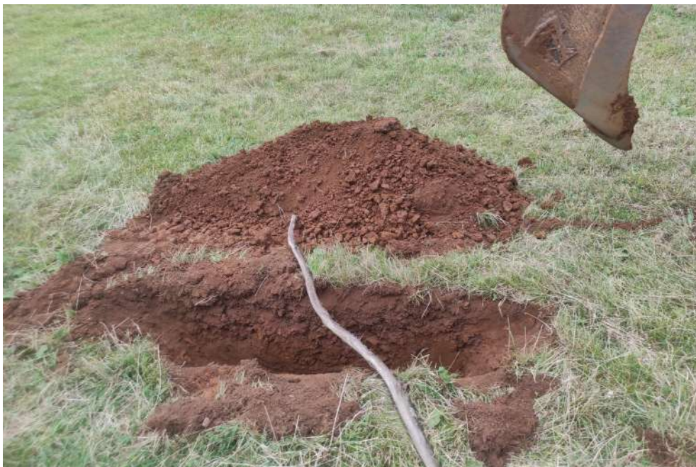
Photograph of arisings from trial pit SA8.
