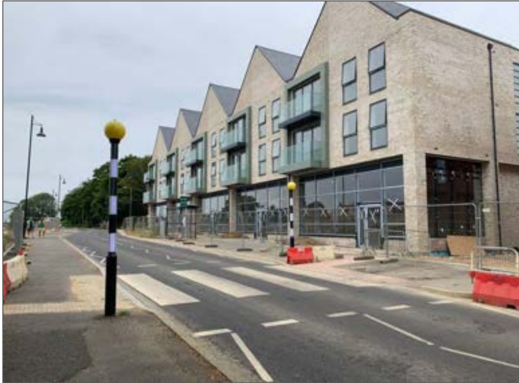
Photograph 4-1 Zebra Crossing on Camp Road
