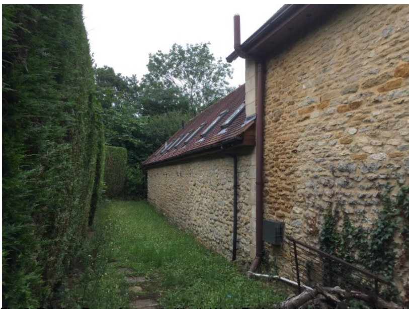
Fig. 2: Existing Rear of property (North-West Facing) with continuous 3.5m high dense Coniferous hedge-row
