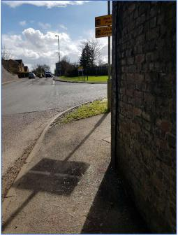
The realigned kerb of the northern exit arm of Bucknell Road, produces a reduced footway width on the western side of the road. The design sketch appears to show a footway width of approximately 1m. The reduced footway width may lead to pedestrians walking in the carriageway to pass others on the footway. This may lead to pedestrian to vehicle collisions. This may be exacerbated by the restricted inter-visibility between opposing pedestrians at this location, due to the railway bridge wing wall.
