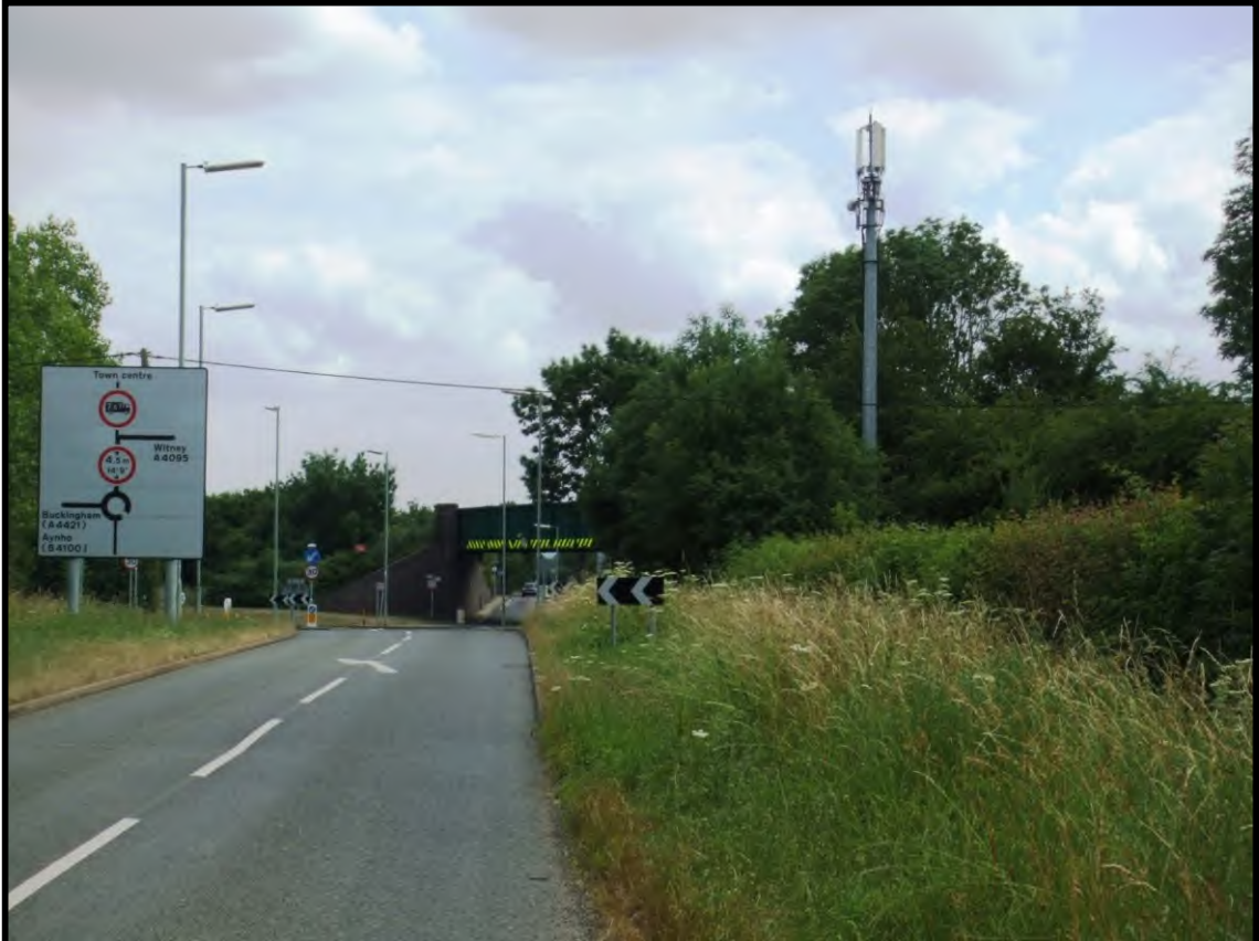
Plate 2: One of four mobile telecommunications masts (all on Messrs. Malins' land). This one is located near the roundabout at Bicester Road and the A4095
