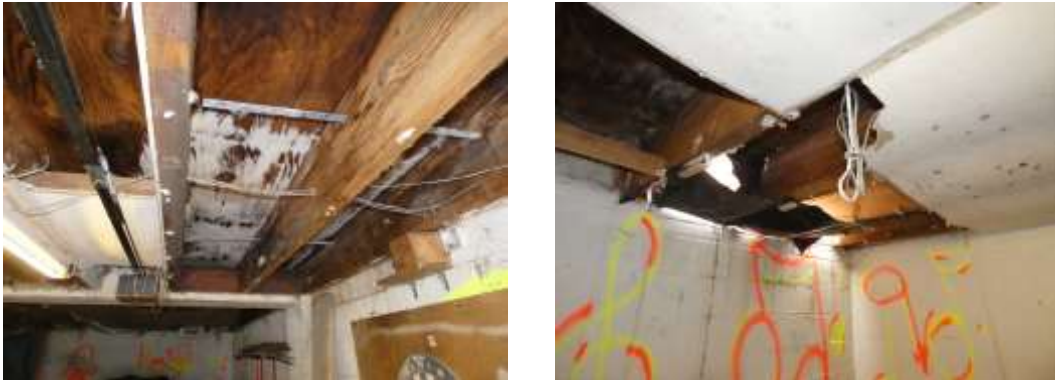
Figs. 13 & 14 Interior of garage
