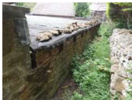
Figs. 5 & 6 Felt covered roof of garage
