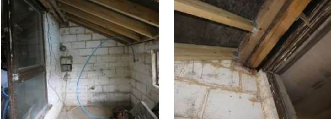
Figs. 17 & 18 Interior of stone lean-to
