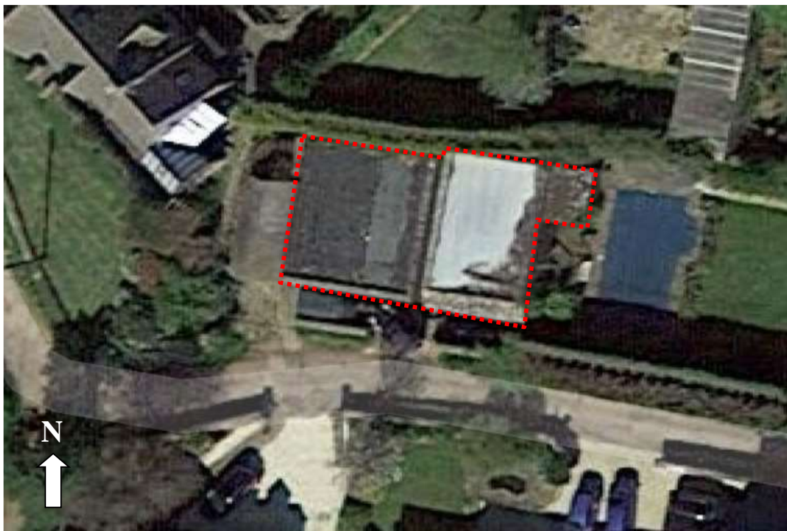
Lane Head garage and store – surveyed building in red outline
