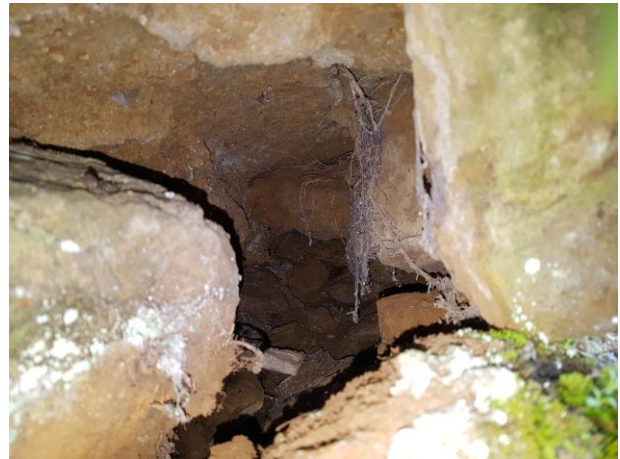
Photograph 8. Interior of a crevice extending into the fabric of the stone walls.
