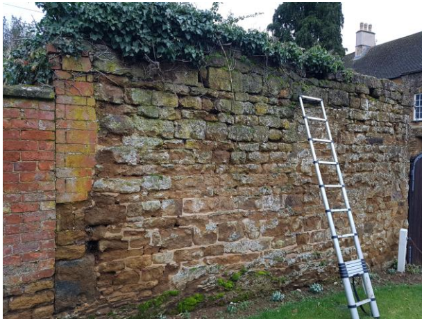
Photograph 7. Missing mortar and crevices on the southern stone walls.
