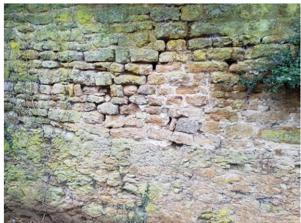
Photograph 6. Missing mortar on the western stone walls bounding the site.
