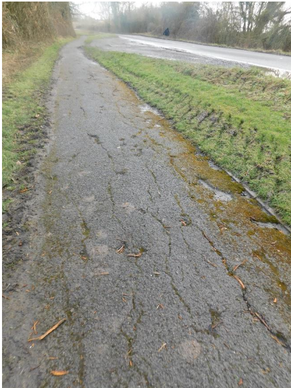
Figure 30: Route 6 - Continued Cracking
