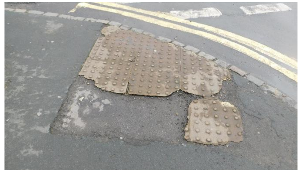
Figure 18: Route 4 - Damaged Tactile Pavings
