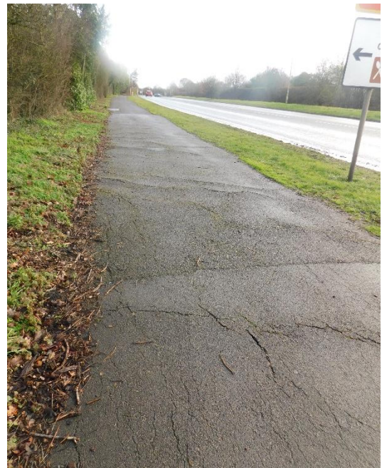
Figure 34: Route 1 - General Conditions and Cracking
