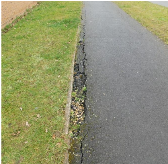
Figure 23: Route 5 - Cracking and Surface Uplift
