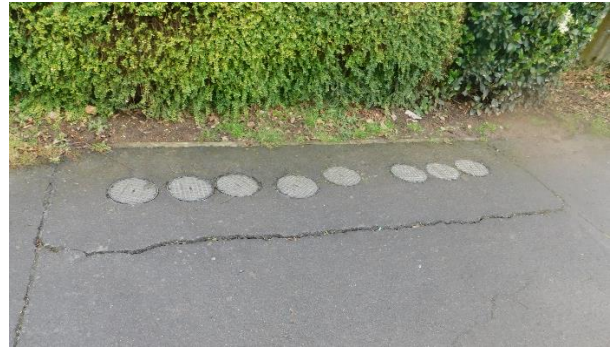
Figure 24: Route 5 - Cracking
