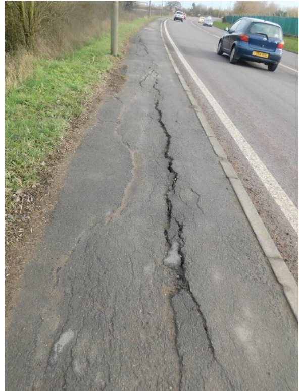
Figure 28: Route 6 - Severe Cracking
