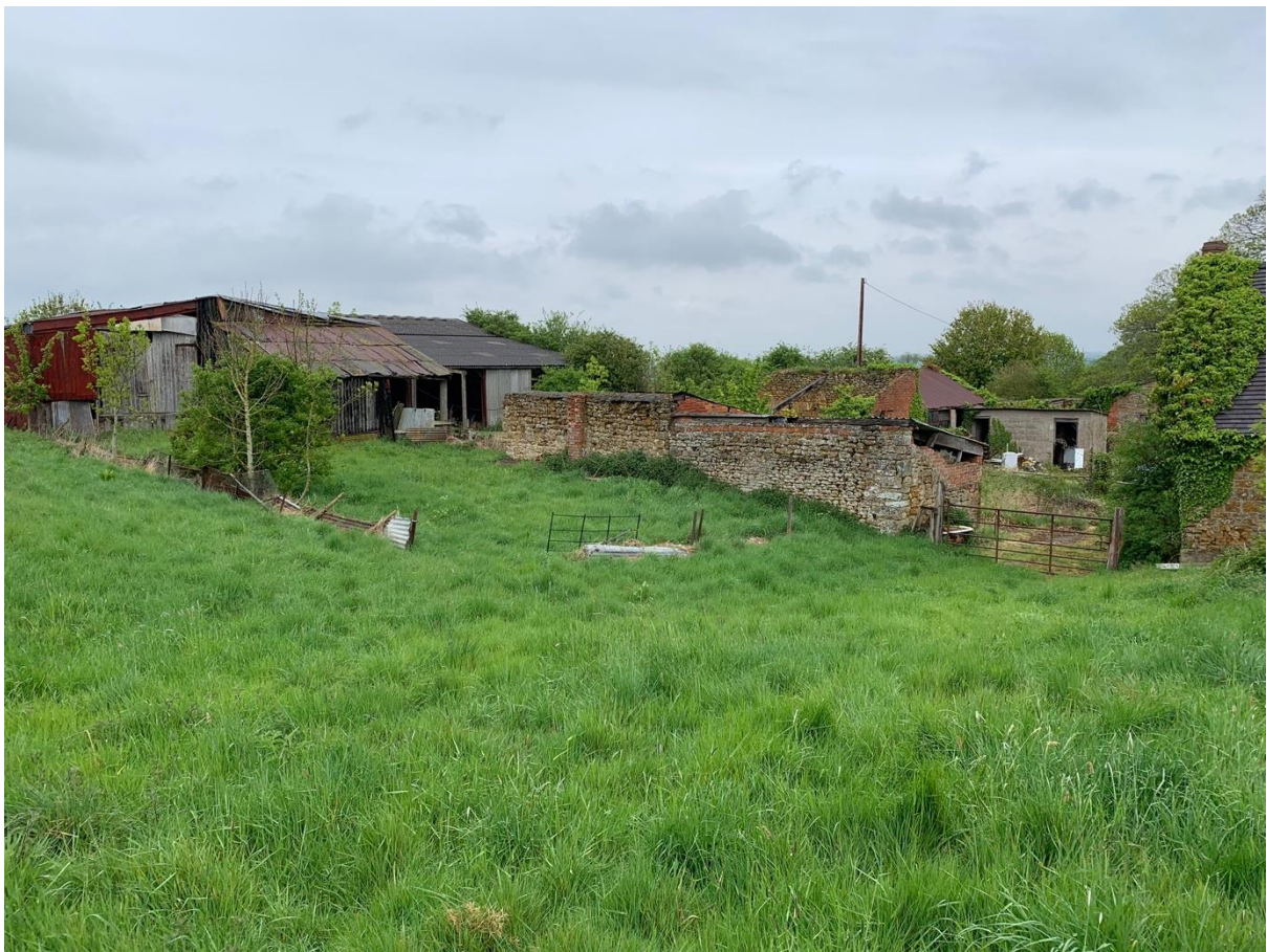
Figure 1: The central area of Crockwell Farm, showing the derelict and disused buildings to be replaced by the new dwellings. The large steel-framed barns to the left do not form part of this application.
