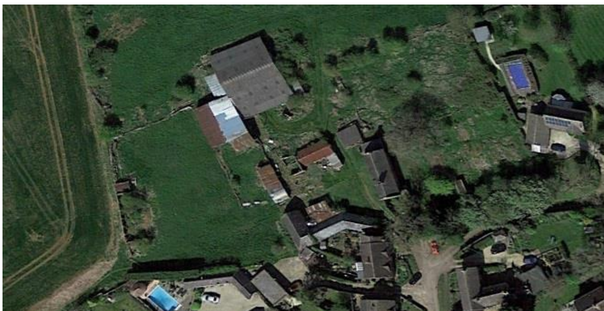
Figure 14: Google Earth images from 2017 shows a further decline in the abandoned outbuildings. Not only has building 6 lost its roof, but building 11 was also completely unroofed and the interior had been invaded by greenery.
