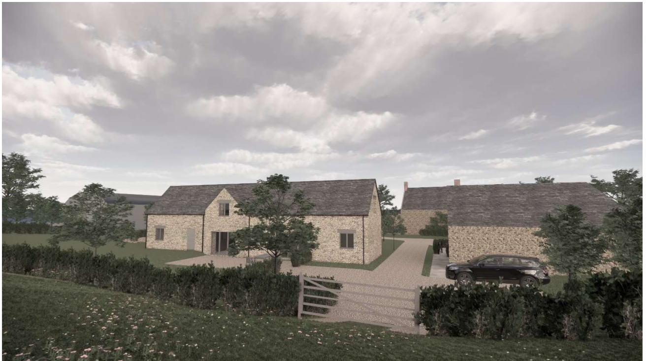
View 2 – Existing Paddock and footpath
