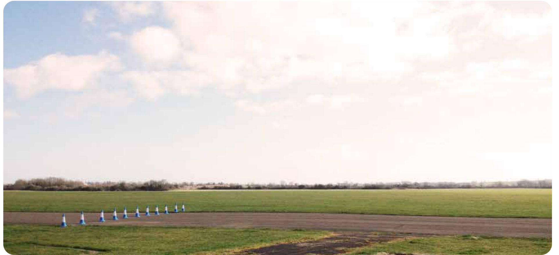
Figure 15. View of Perimeter Track
