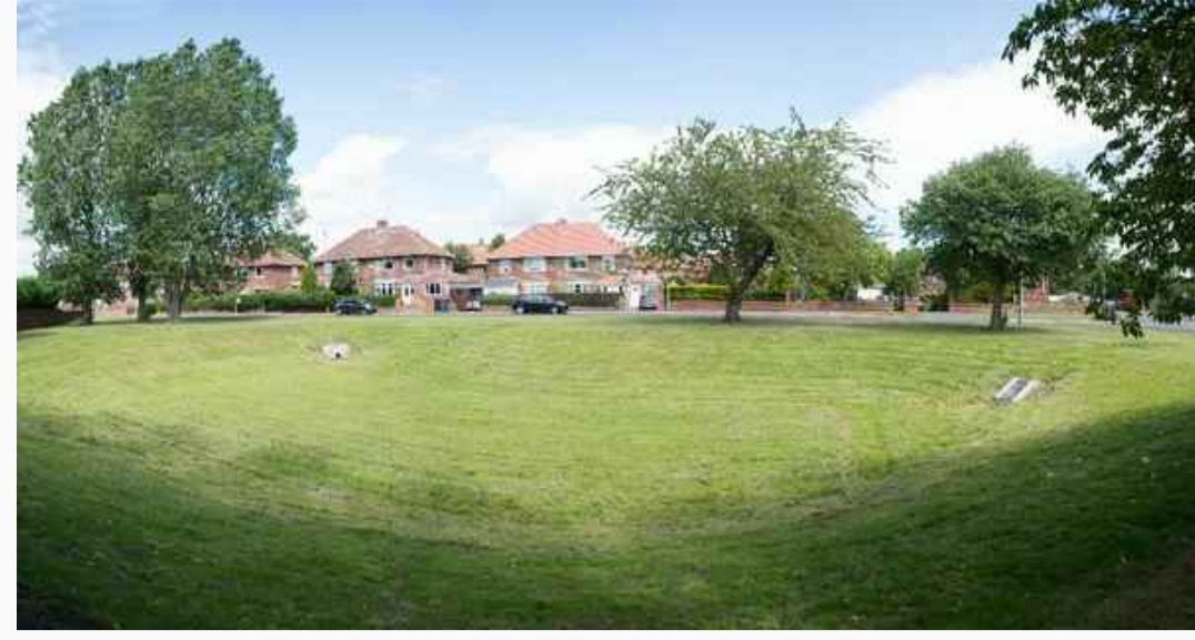
IMAGE 2 - TYPICAL EXAMPLE OF AN INFILTRATION BASIN
