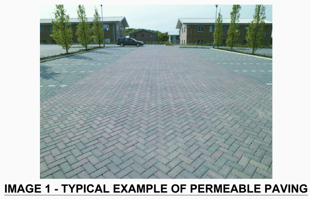
IMAGE 1 - TYPICAL EXAMPLE OF PERMEABLE PAVING
