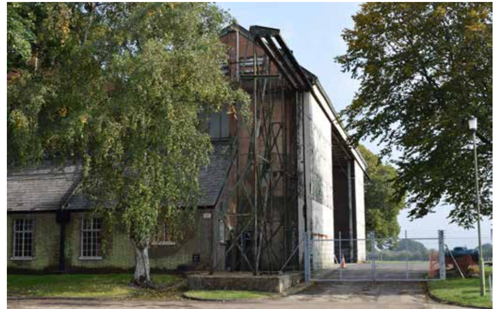
Fig 30: Southern most Type A Hangars
