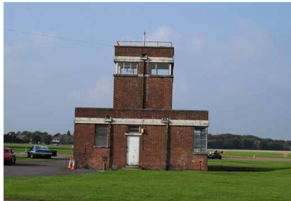
Fig 9: Watch Tower at RAF Bicester. The base stands out in its continued use of brick - with the latter material used even in the construction of early wartime additions such as the Bomb stores. This is thought to have been driven by recommendations made the Royal Fine Art Commission with the aim of maintaining the 'aesthetic coherence' of the base.
