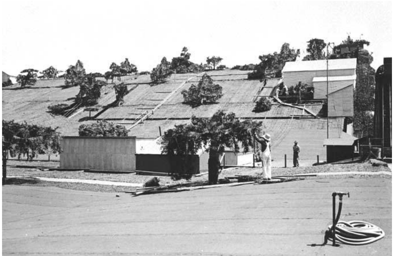
A3: Fig 6: WWII Airbase factory in California covered in camouflage netting.
