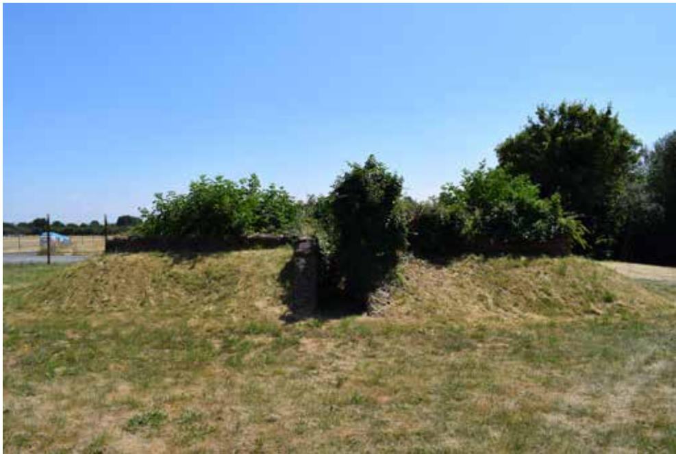
A3: Fig 8: Earth Traversed shelters at RAF Bicester
