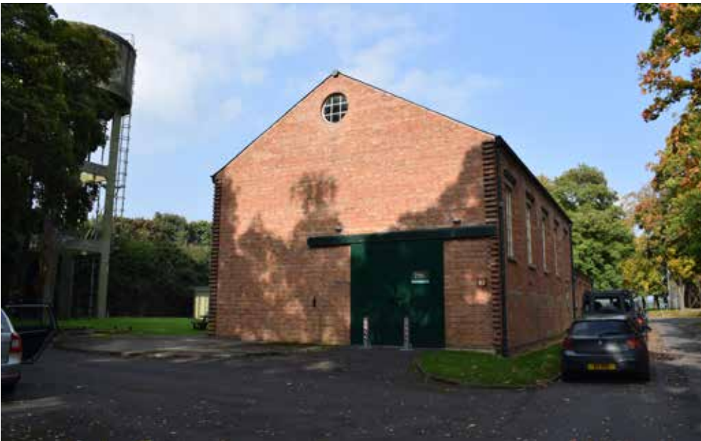
Fig 26: The Parachute Stores. The design of the building - featuring a high central area- is particularly informed by its function. The Stores at Bicester were a prototype, first seen here before being adopted in airfield sites elsewhere across the country.
