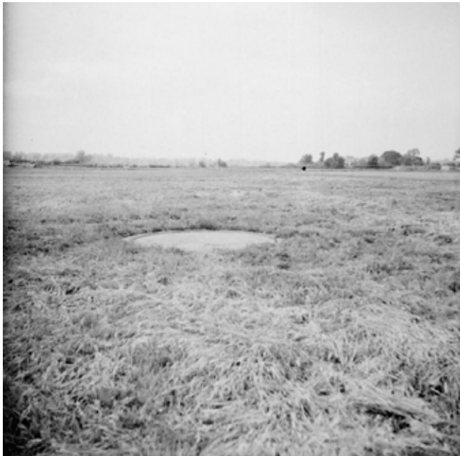
Fig 17: Retractable ‘Pickett-Hamilton’ pillbox in closed position on a grass airfield. The structure was designed to optimise the element of surprise in the event of an invasion. Speed was therefore of the essence. The initial lifting mechanism used to raise the inner cylinder - originally consisting of an 8-ton aeroplane jack - proved rather slow (taking 3 minutes to open). It was later replaced with a pneumatic ram operated with compressed air that allowed for the structure to be raised more quickly.
