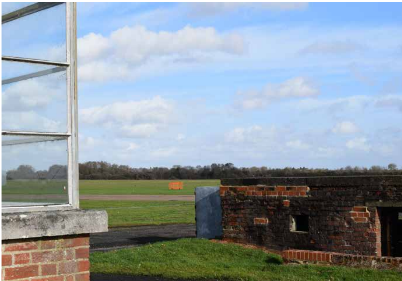
Fig 43: View across the airfield from the base of the watch tower.
