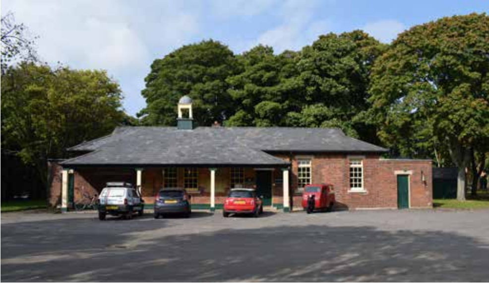
Fig 25: The Guard house, prominently sited at the entrance of the site and built in a neo-Georgian style thought commensurate with the activities carried out with it and with the status of its occupants.
