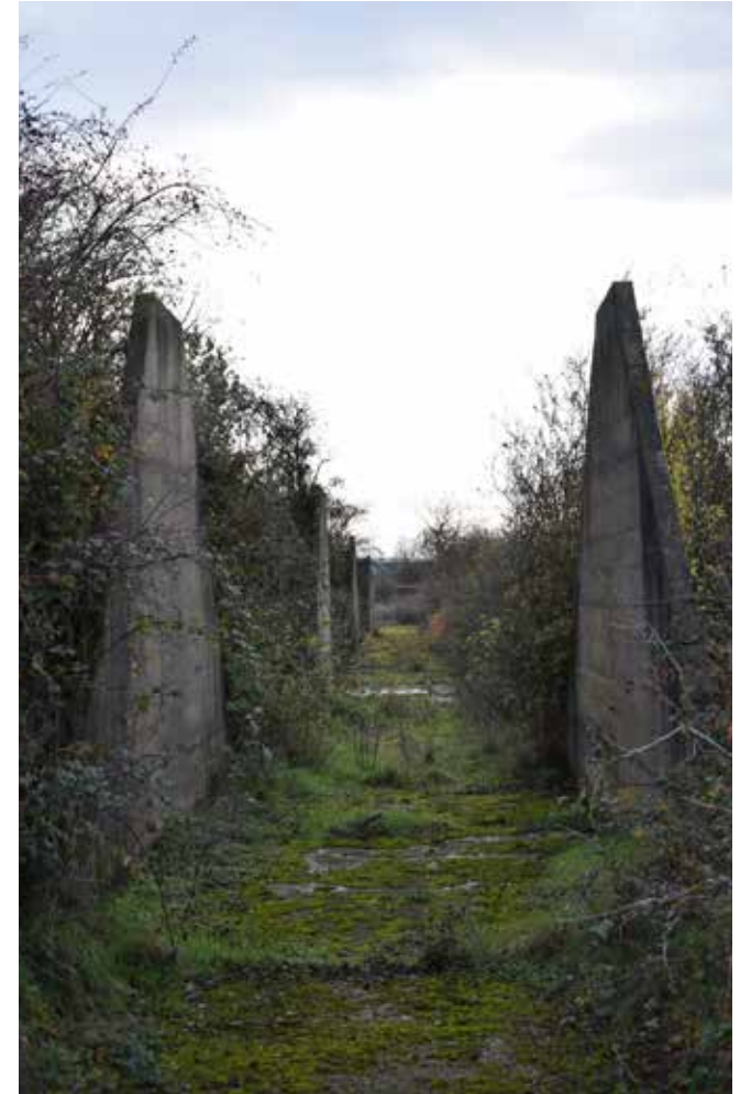
Fig 45: View of the bomb stores showing the earth banks and the gantry.
