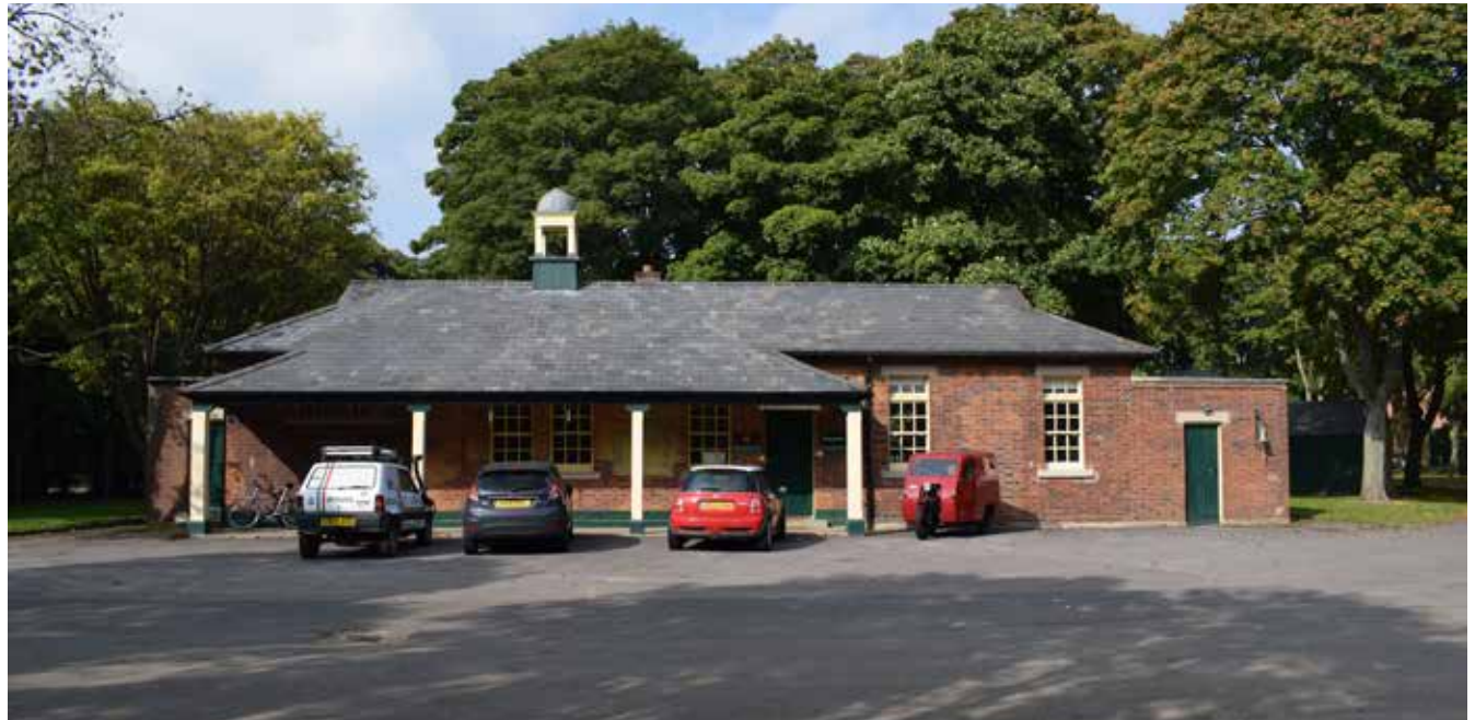
A3: Fig 5: The Guard House at RAF Bicester. The building, prominently sited at the entrance of the site, is of a neo-Georgian style and in colours typical of the time; constructed of 'earthy' red brick with a grey slate roof and green wood finishes.
