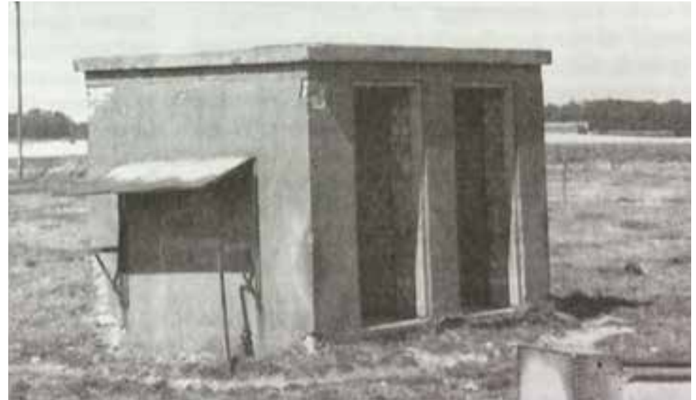
Fig 14: Example of a 'Ready Use Pyrotechnic Store at Ingham c1983 (Francis 1996: 53)
