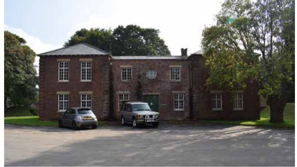
Fig 27: The Station Offices and Headquarters. Situated directly opposite the Guardhouse, the application of the neo-Georgian treatment to its design is also meant to symbolically emphasise the status of its occupants and serves as a strong visual marker of the relationship between the two buildings.
