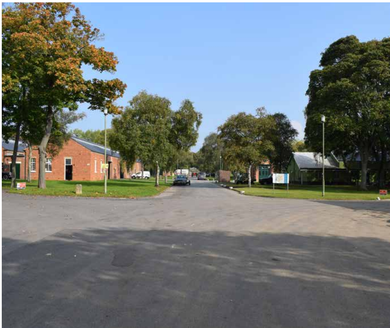
Fig 7: View looking east through the centre of the Technical Site'
