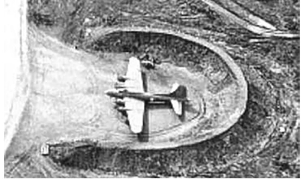
Fig 54: Blast revetment around a panhandle
