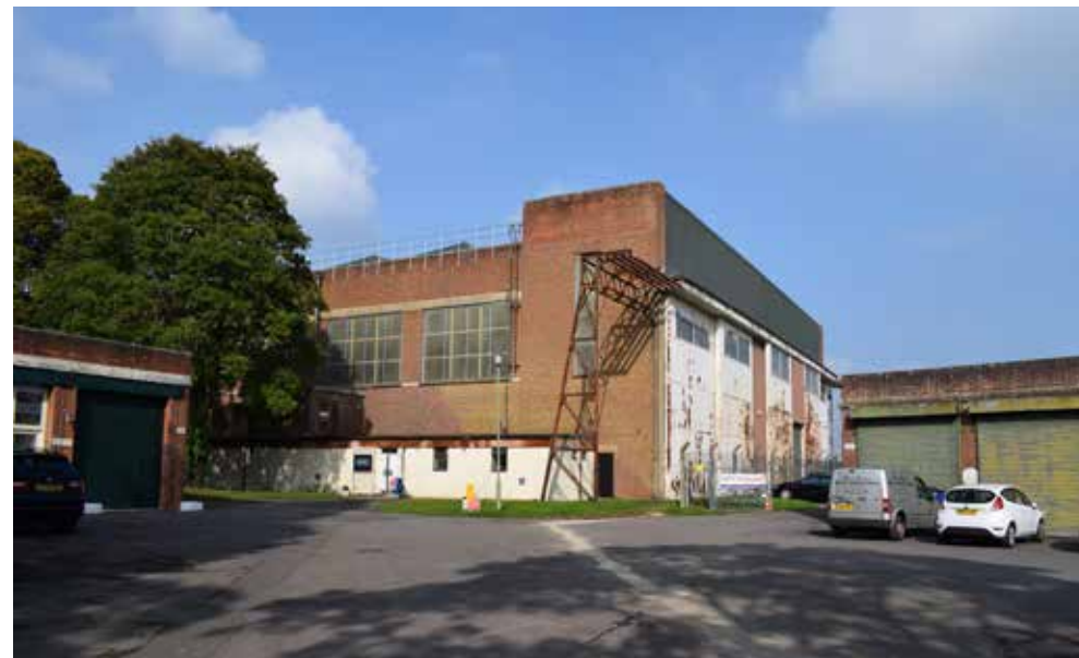
Fig 33: Northern most C Type Hangar
