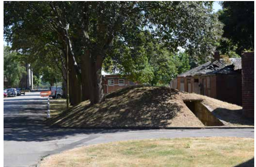
A3: Fig 9: Earth Traversed shelters at RAF Bicester
