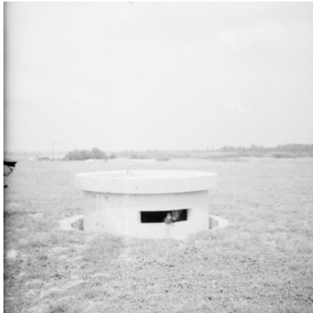
Fig 18: Retractable ‘Pickett-Hamilton’ pillbox fully raised. Once open the pillbox could be operated by two men. Such defences were largely constructed during the ‘invasion crisis of the early war years (1940-1941).
