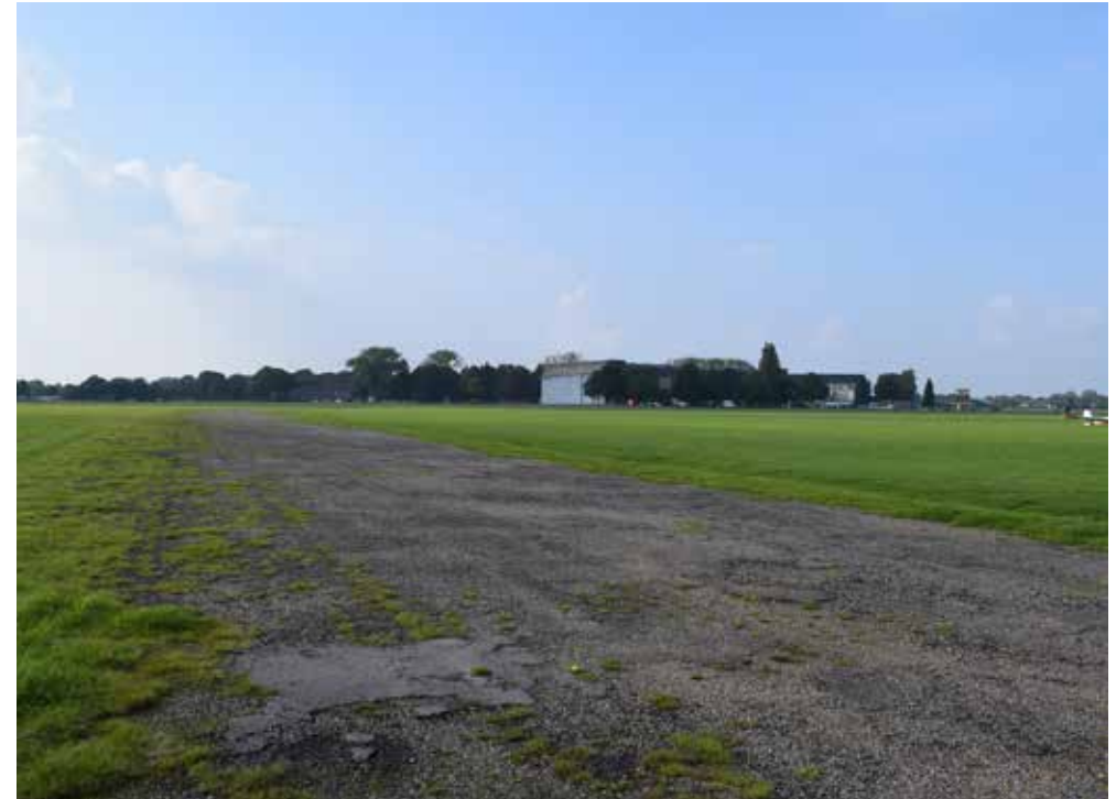
Fig 11: View of section of the Perimeter Track at RAF Bicester. The track was tarmacked but with an asphalt finish to help camouflage the area
