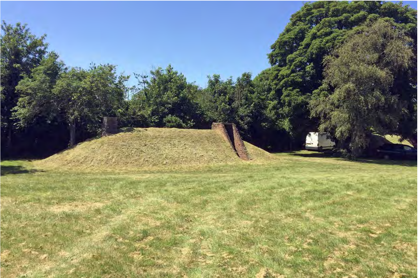
Plate 9: Detail of central air raid shelter
