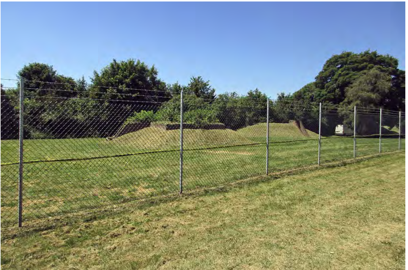
Plate 8: Air raid shelters to the south of the technical site
