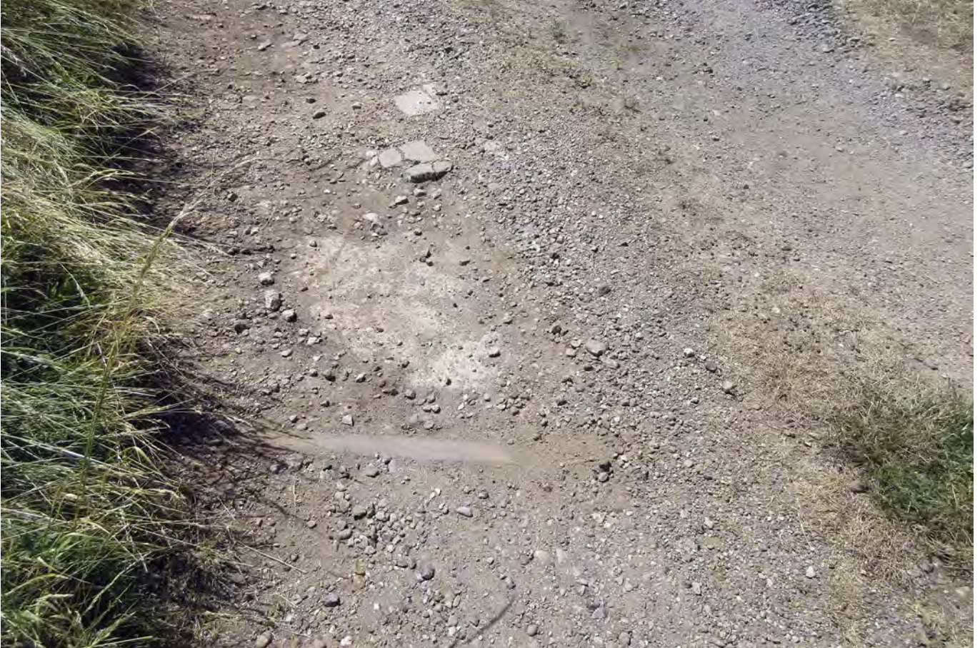
Plate 17: Surviving in-situ railway line observed in the south-eastern corner of the site
