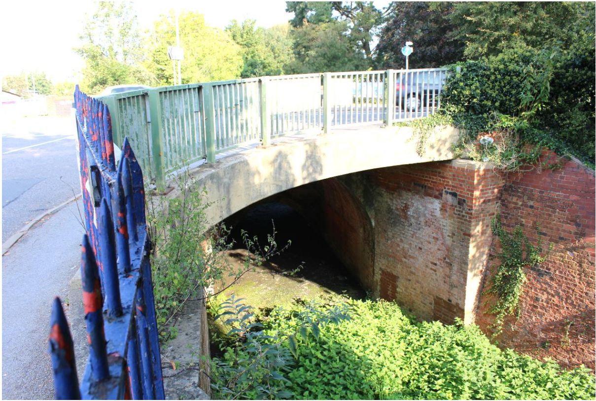
Image EDP 4: Grade II listed Bridge over Mill Stream ( 1046184 ) from south, showing limited experience of the stone medieval structure encased in later alterations.
