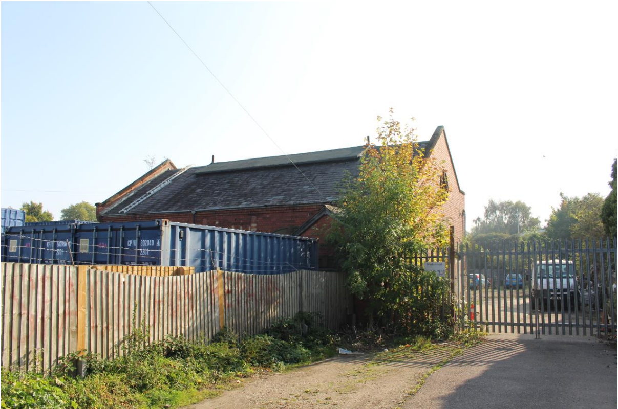
Image EDP 9: Vacant Former British Waterways building (NDHA3), looking east.
