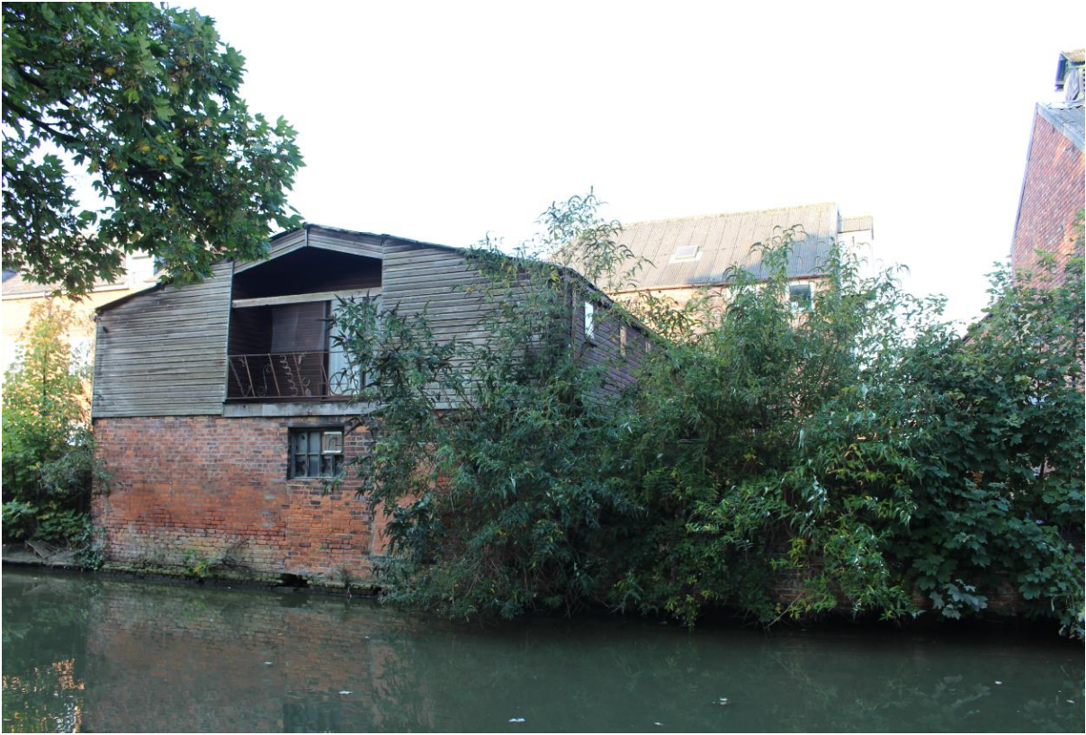
Image EDP 8: Canal-side elevation of Corporate Printers building (NDHA2), looking east.
