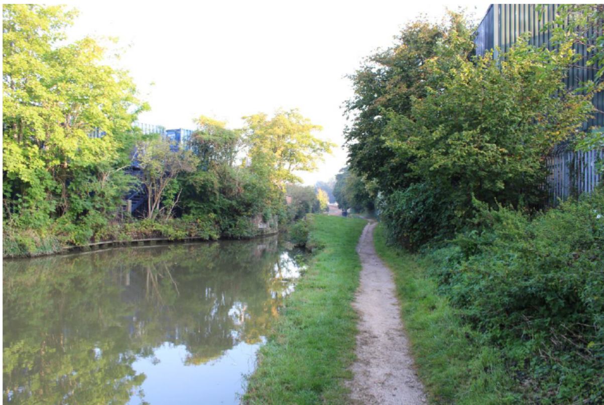
Image EDP 6: View north along the Oxford Canal Conservation Area, within the section to the south of Bridge Street. Note the enclosed character, with views tightly channelled along the waterway.
