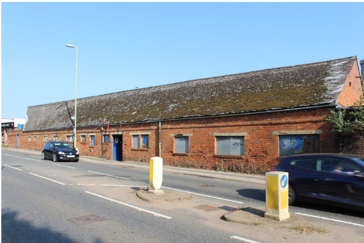
Image EDP 11: Laser Sailcraft building (NDHA5), looking north-west.
