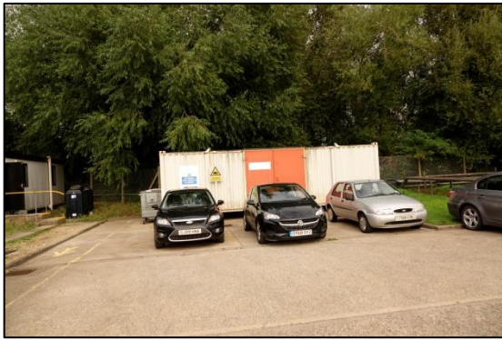
Photograph 9: Buildings within the Site
