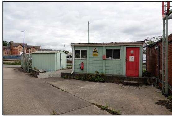
Photograph 10: Buildings within the Site
