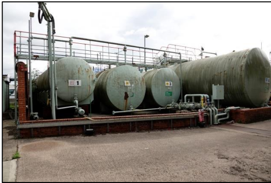
Photograph 11: Buildings within the Site
