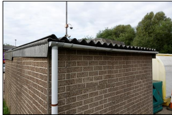
Photograph 12: Buildings within the Site
