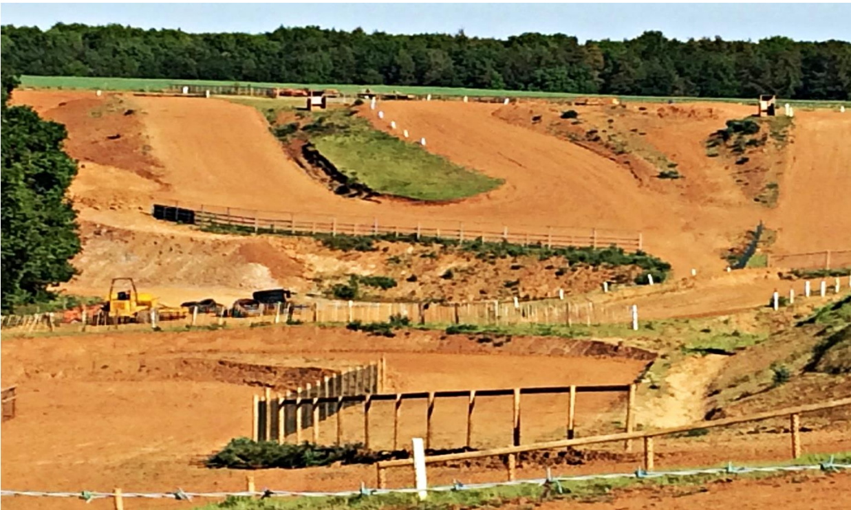
New earthworks reaching completion – diggers still present. Image taken 28 May 2020.
