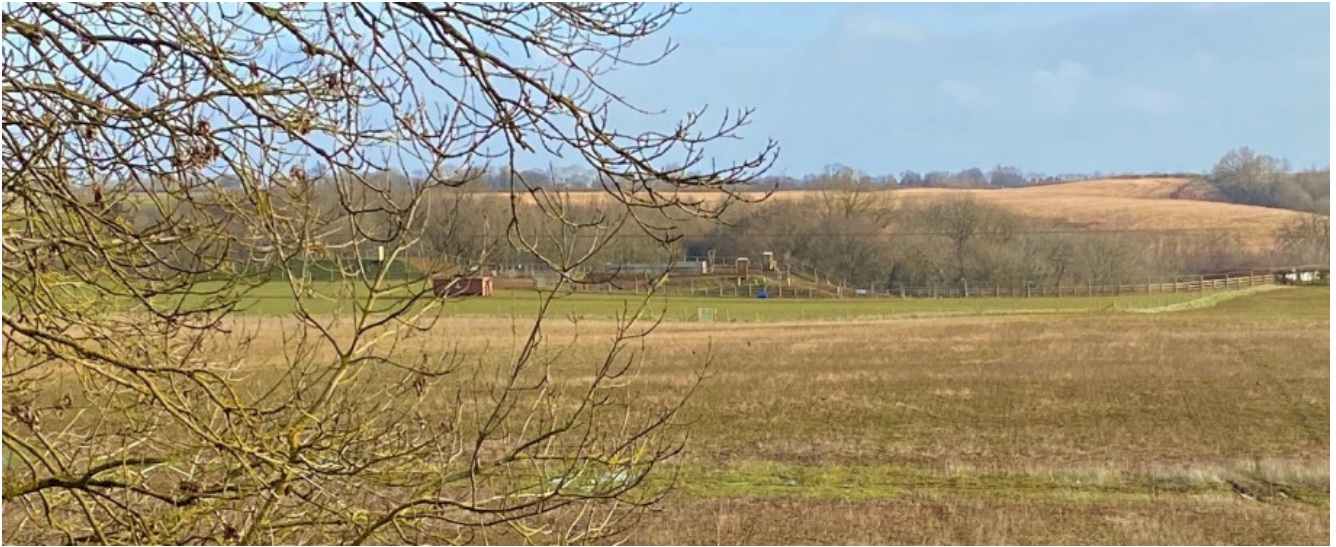
Shot taken with iPhone from A422 March 2021, with skip, marshal hut etc clearly visible.
