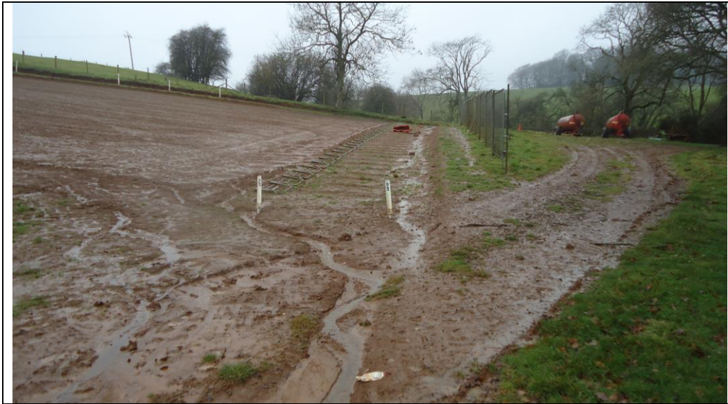
Plate 9: Looking west at the north west corner of site (circuit starting line) showing rills formed in the exposed soil and run-off following the track in the foreground, eventually entering the watercourse
