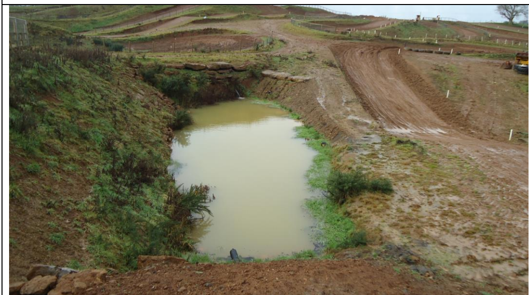
Plate 6: Looking east across pond (TN6) which is used as a silt trap.
