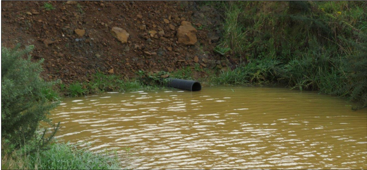
Figure 15 Outflow from the upper pond, set at the pond's eastern end
