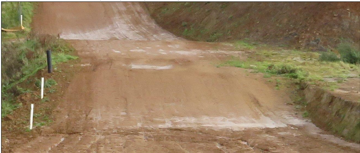
Figure 26 Water accumulates temporarily in low points along the track
