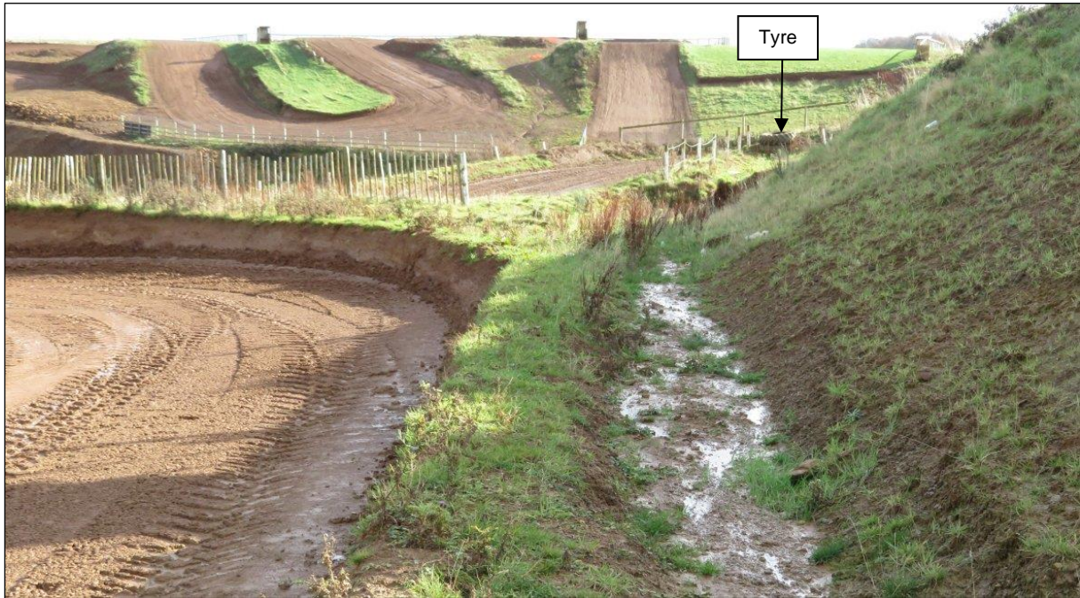
Figure 23 A swale located at the base of a slope, excess runoff is conveyed towards the tyre and piped to the upper pond
