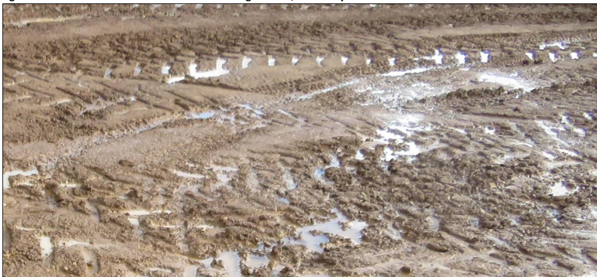
Figure 27 Water accumulated in small surface irregularities, such as tyre tracks
