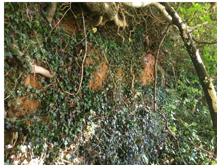
Plate 5: South face of the bank at the northern boundary of the site
