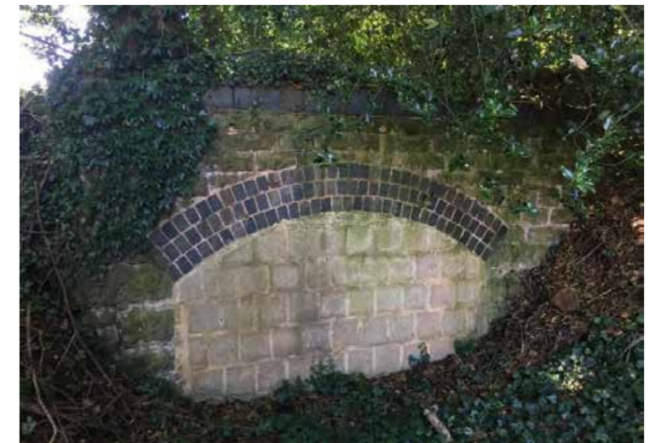
Plate 8: Close-up of infilled subway arch in the south-western corner of the site
